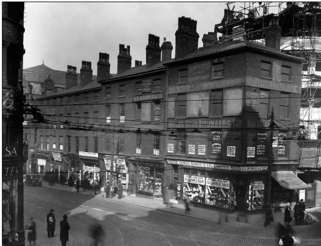
Plate 12: Blackfriars Street, looking north-west from Deansgate, 1933
