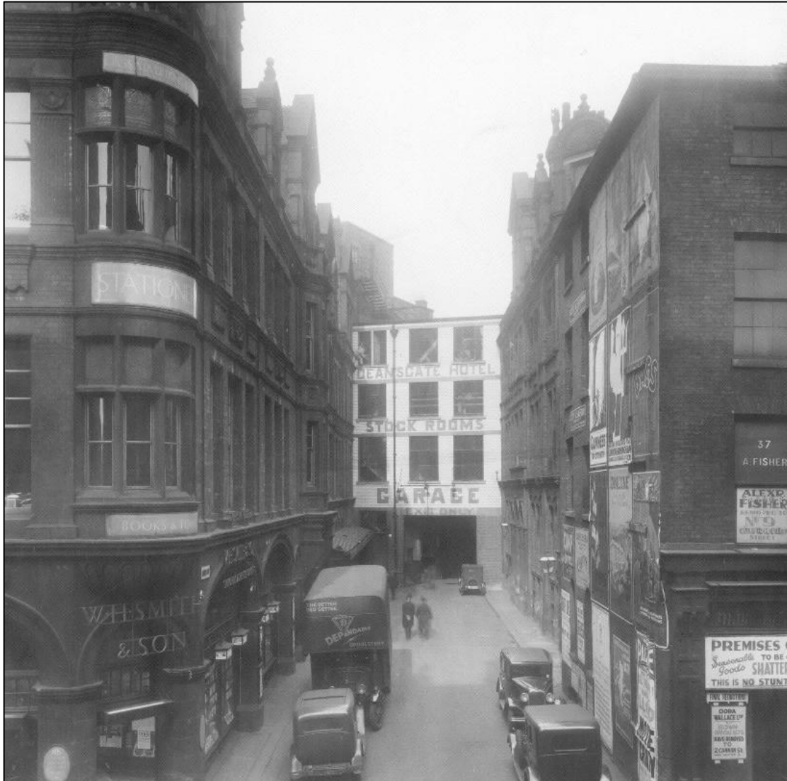
Plate 13: Photographs of Carr Street, looking north from Blackfriars Street, 1933
