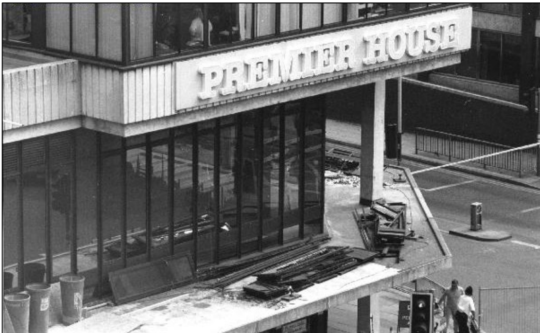
Plate 18: Damage from 1996 IRA bomb, Premier House, Deansgate (West side), corner with Blackfriars Street, Manchester
