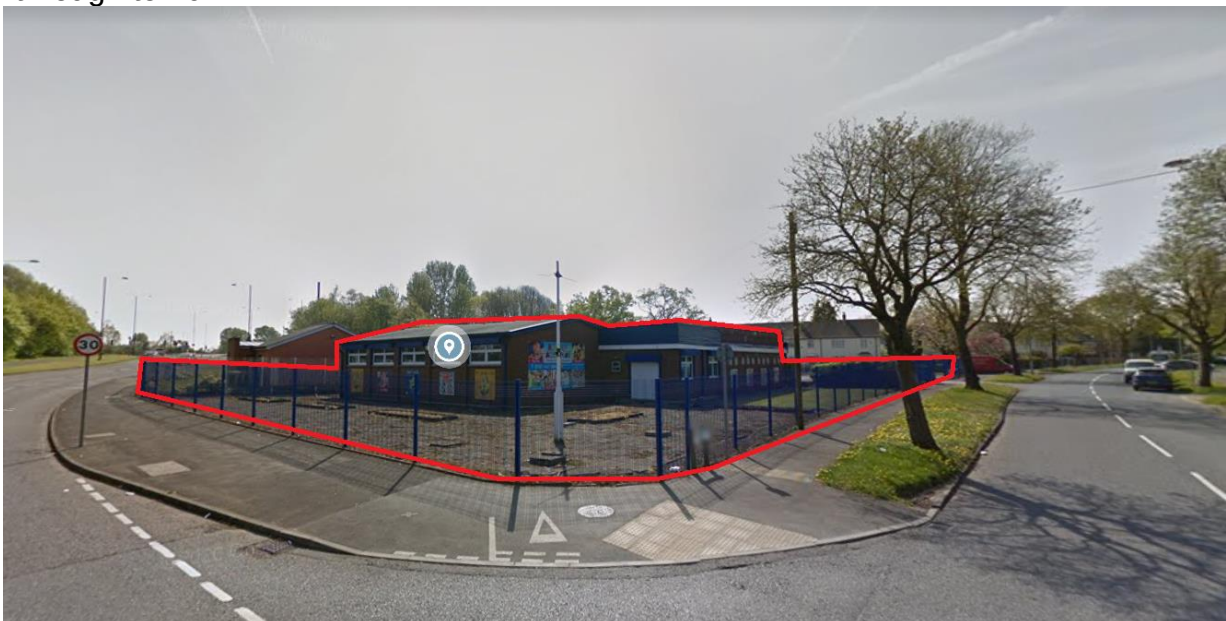
Application property and demise
