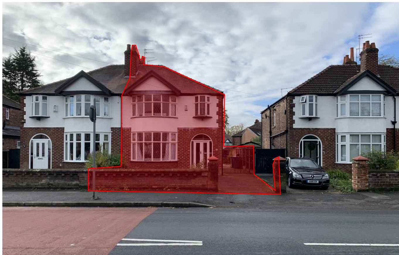
Photograph 1 Application site as viewed from Fog Lane
