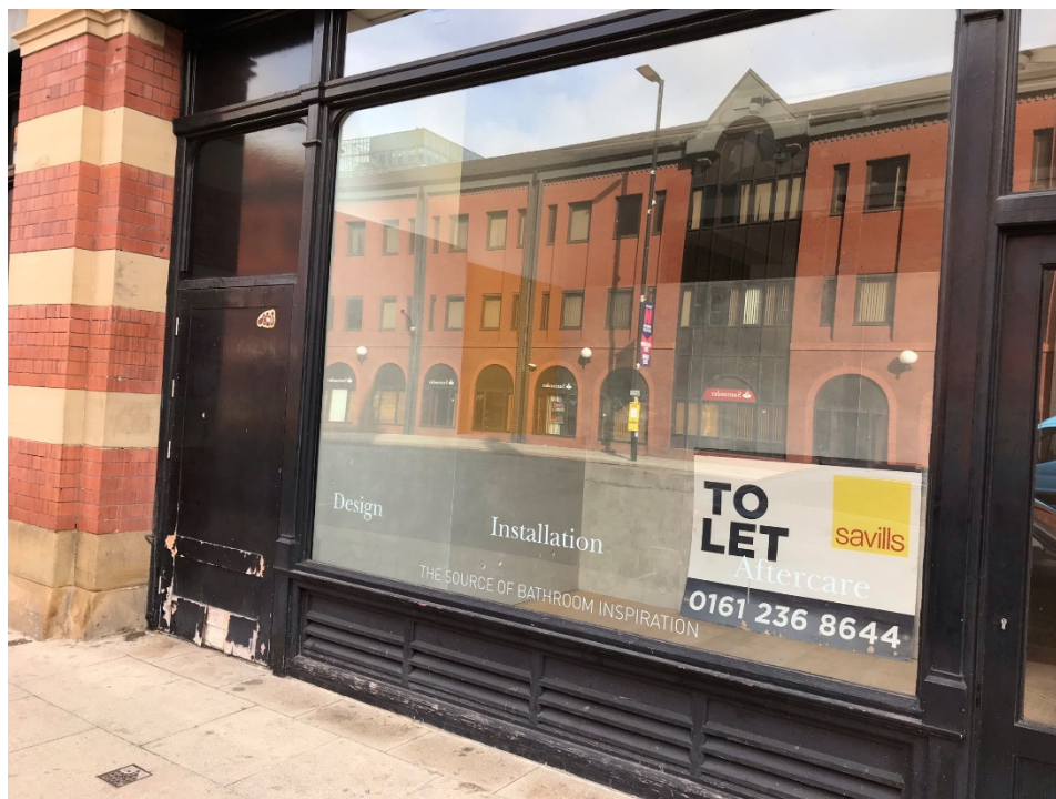
18. External view of Unit 265.
