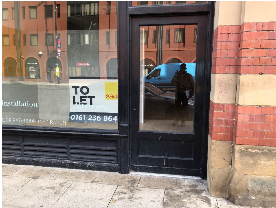
19. External view of Unit 265.
