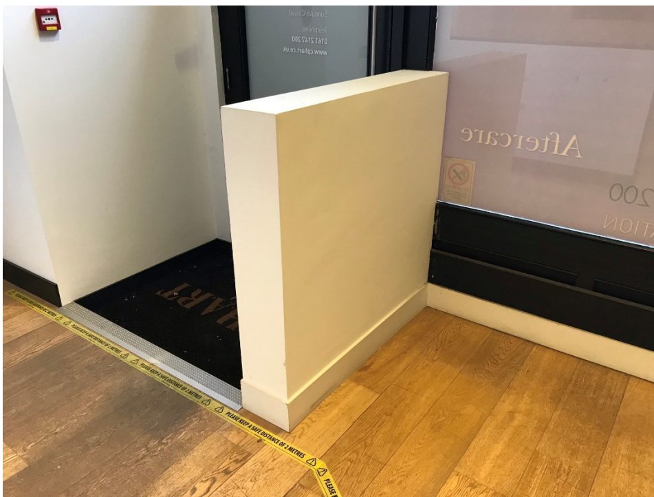
4. Area of proposed access ramp, existing partition to be removed to accommodate the ramp.
