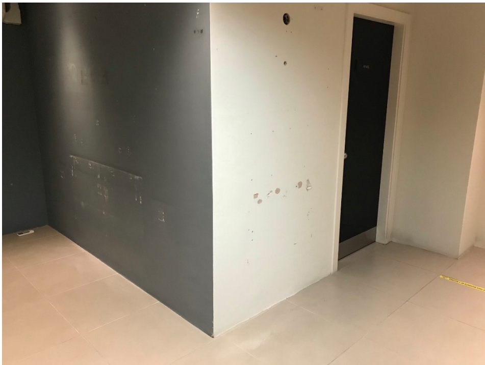
8. General view of basement to Unit 265. Existing partition to remain.
