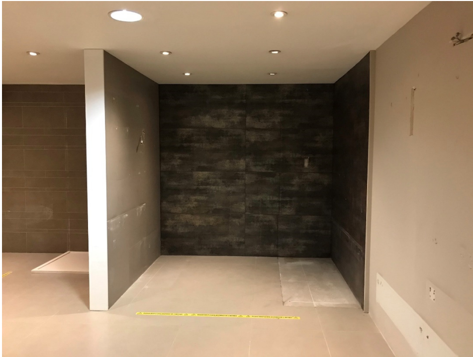
7. General view of basement to Unit 265.
