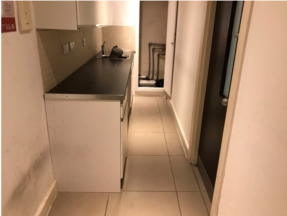
15. General view of existing kitchen to Unit 261, to be retained.
