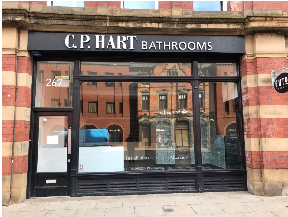
17. External view of Unit 267.
