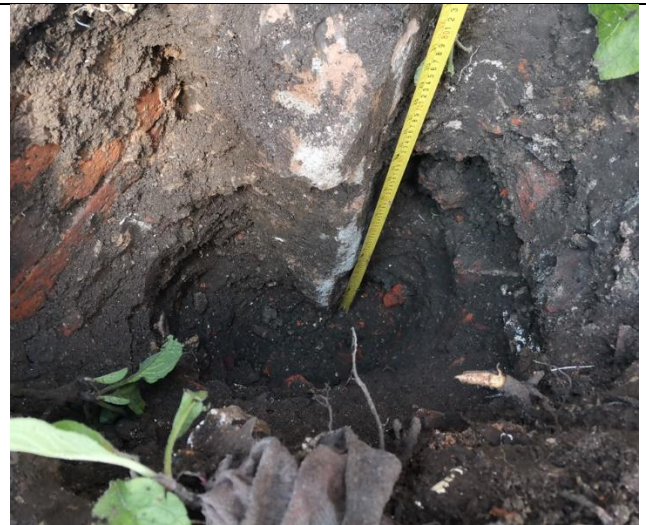
Trial Pit 02: Internal view of excavation
