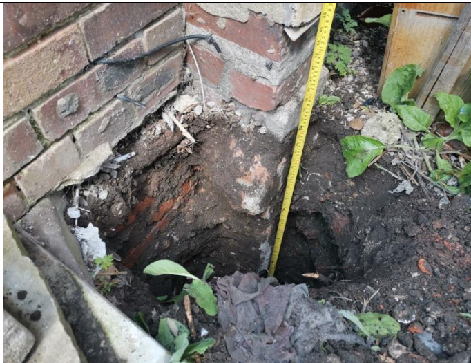
Trial Pit 02: Overview of excavation
