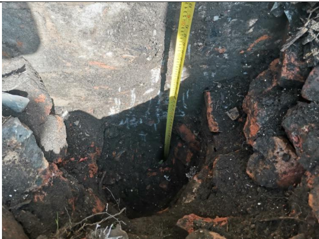
Trial Pit 01: Overview of excavation
