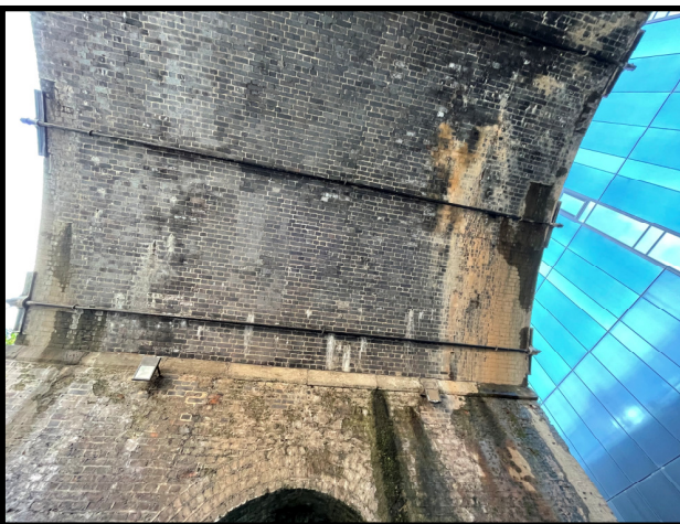
Plate 4 The brickwork is generally in good condition
