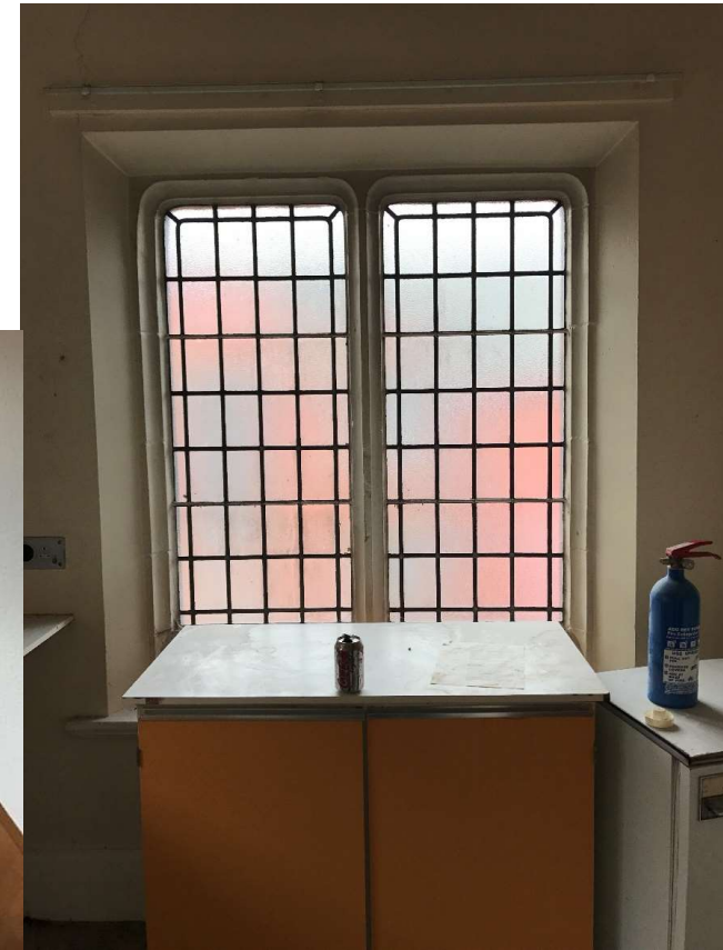
Original windows with ornate detailing
