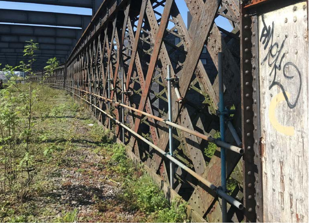
Photo of existing scaffolding poles
