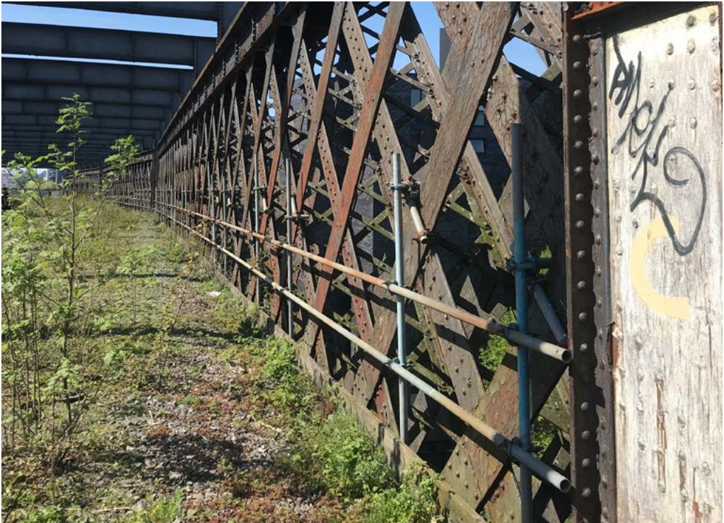
Photo of existing scaffolding poles
