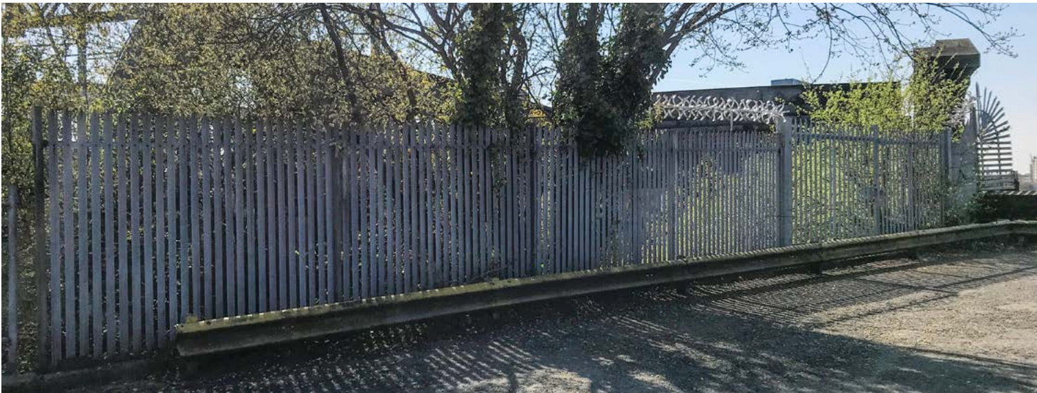
Photo of existing palisade fence and gate
