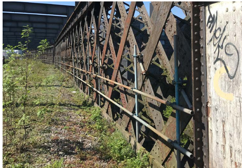
Photo of existing scaffolding poles
