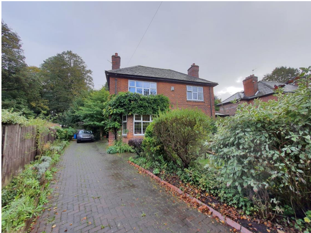
61 Kingston Road – front view as existing
