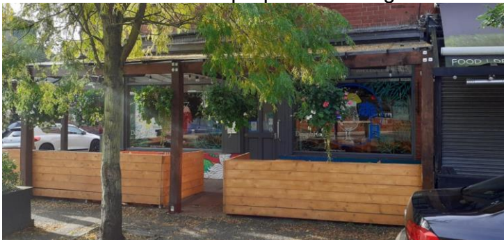
Unauthorised canopy to east
