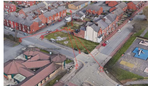
The focal point of the area
