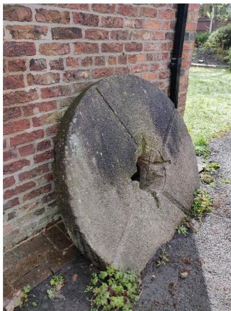
Millstone in its current, inappropriate location on the West elevation of the property
