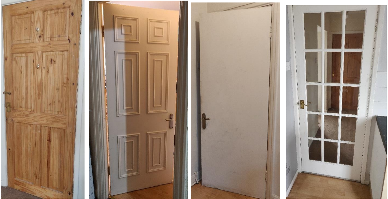
Current doors in property, none of which are original and different styles are seen between the two flats.
