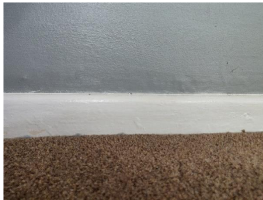
Three examples of the different types of skirting boards found throughout the property. All are of shallow, more modern profiles so aren't believed to be original.
