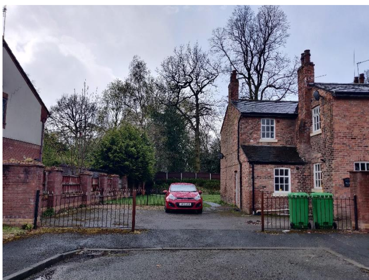
Current driveway condition alongside railings which require restoring.
