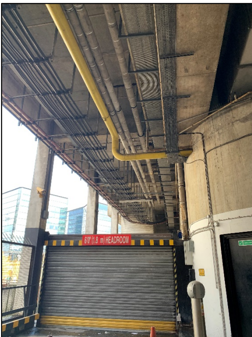
Photo 11 Example of service yard construction
