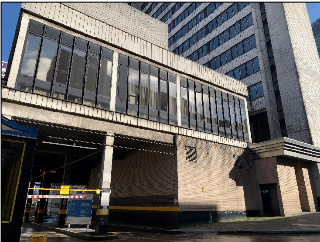
Photo 3 Concrete construction of building
