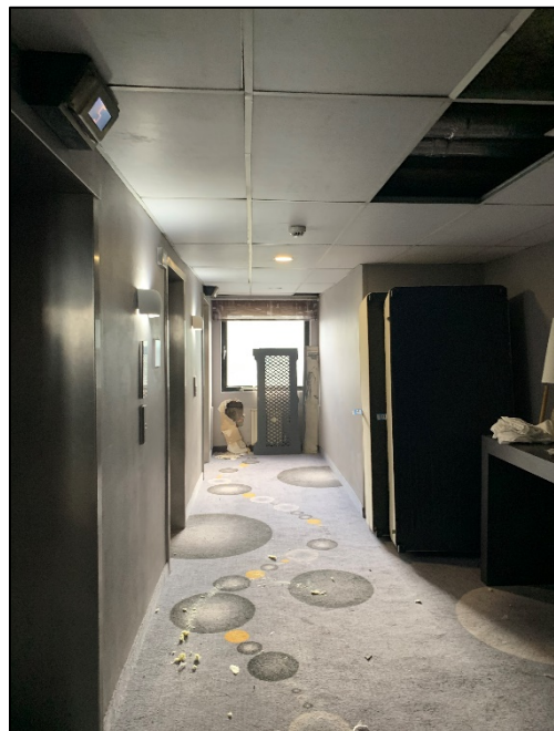
Photo 12 Example of internal aspect of the structure
