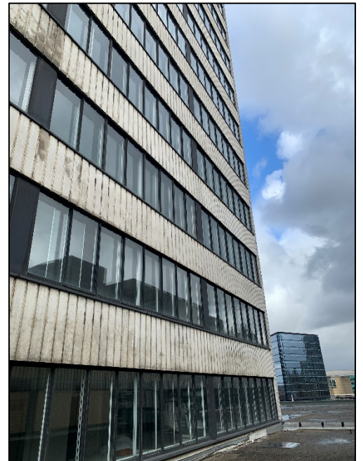
Photo 4 View of hotel 13-storey tower from second floor window
