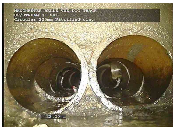
UP_STREAMX_353912d8-0d2d-4ea4-b3c5-a4e89d10e7c9_2 0211014_095353_969.jpg, 00:08:12, 22.20 m General remark, SPLITS INTO TWO 150MM PIPES
