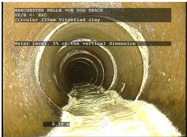
UP_BX_4d9fa507-f3b1-406c-9075-88eeae661ec_20211115_102318_365.jpg, 00:00:06, 0.70 m General photograph taken at this point
