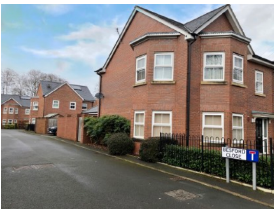
Besford Close - A development of family housing in Fallowfield, built by Watkin Jones in 2013
