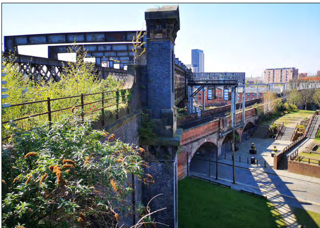
Figure 1.1: Existing Viaduct Structure (source: The National Trust)
