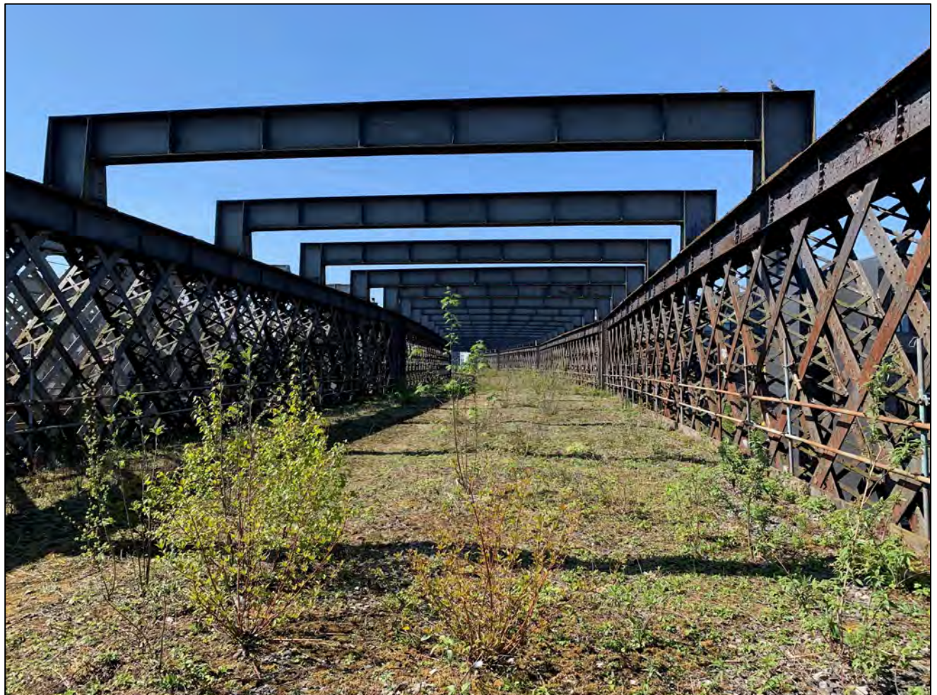
Figure 2.1: Existing Viaduct (source: The National Trust)
