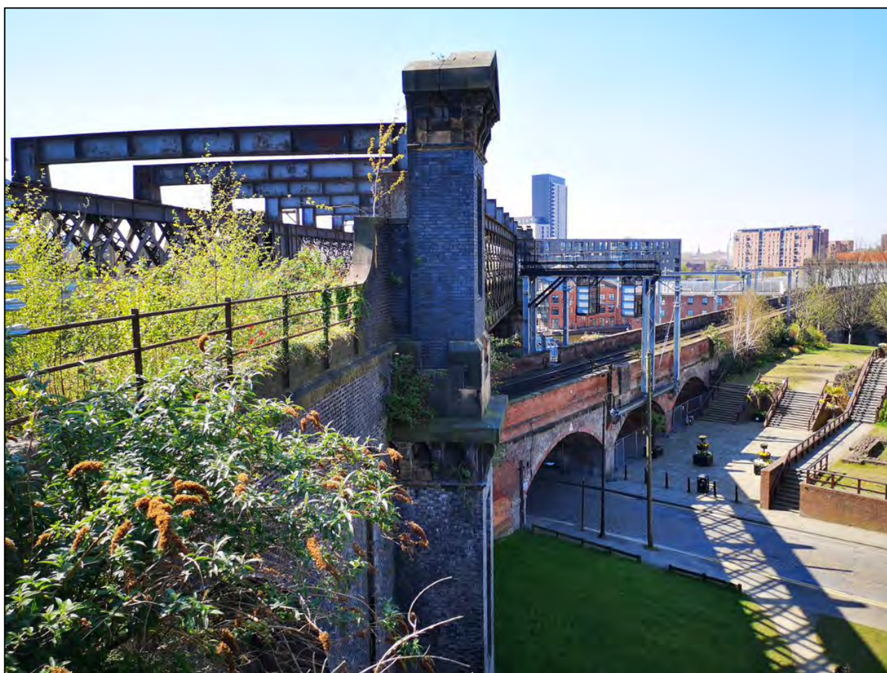
Figure 1.1: Existing Viaduct Structure (source: The National Trust)
