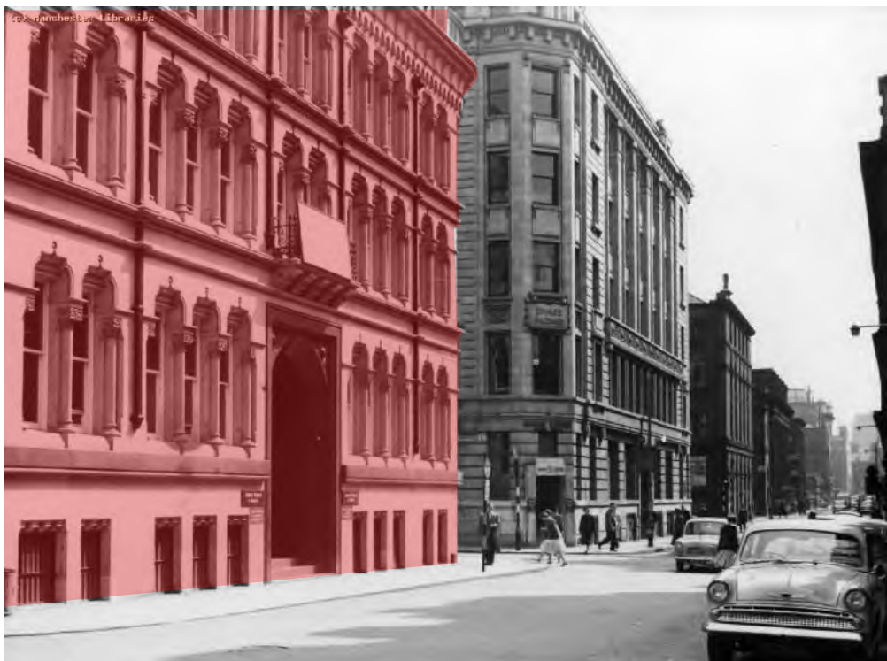
Figure 12: Historic Image c.1960s: The Site at 49 Spring Gardens is indicated in red. The image illustrates the buildings streetscape context during the mid-20th century, which was defined by the Danlee Buildings (now demolished) to the immediate east.
