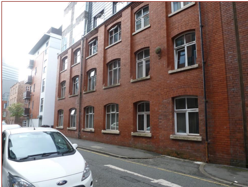
Photograph 01 - View along Simpson Street showing the South-eastern Elevation
