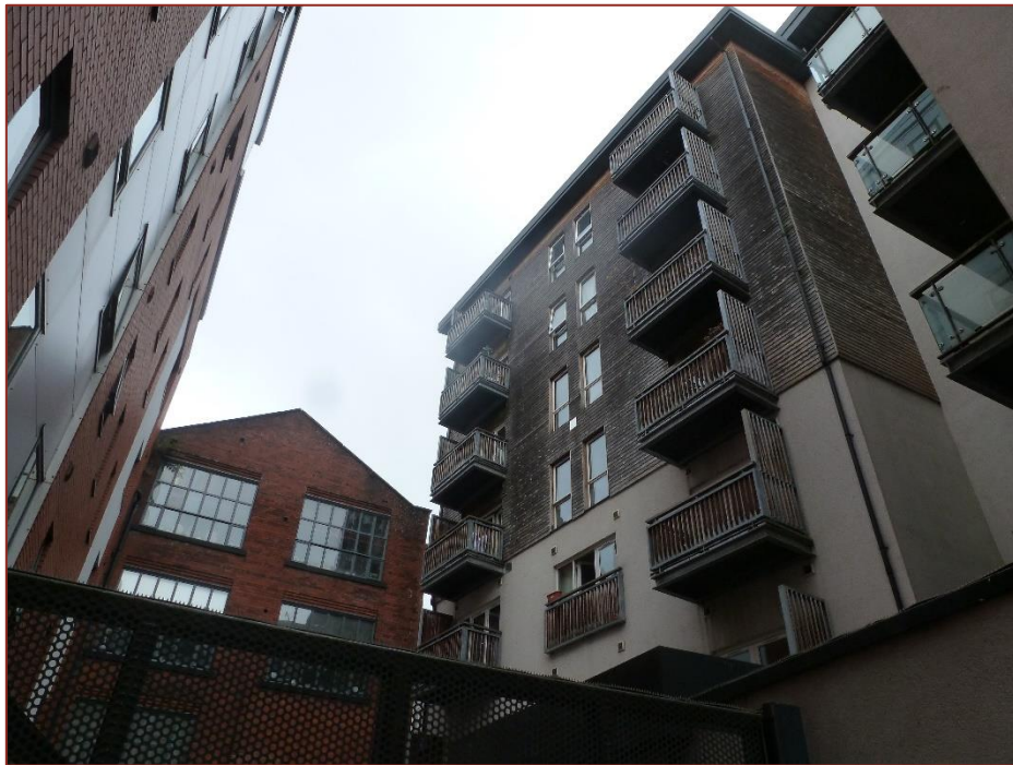
Photograph 04 - Western Elevation of the new build part to the rear of the original building
