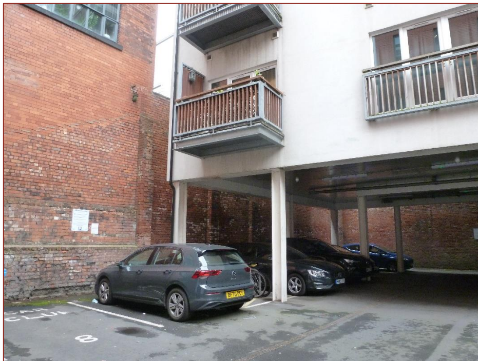
Photograph 05 - Western side of the under-croft car park
