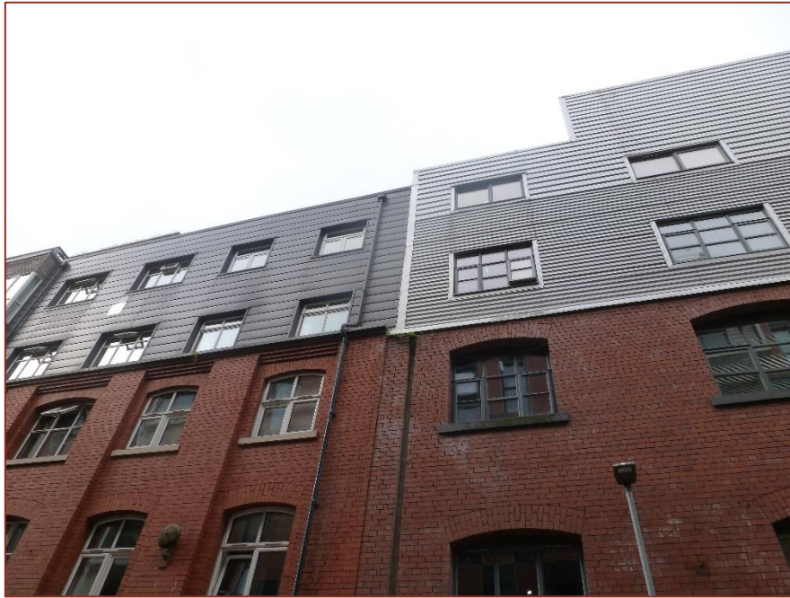
Photograph 02- South-eastern Elevation showing joint between the adjacent building to the right-hand side
