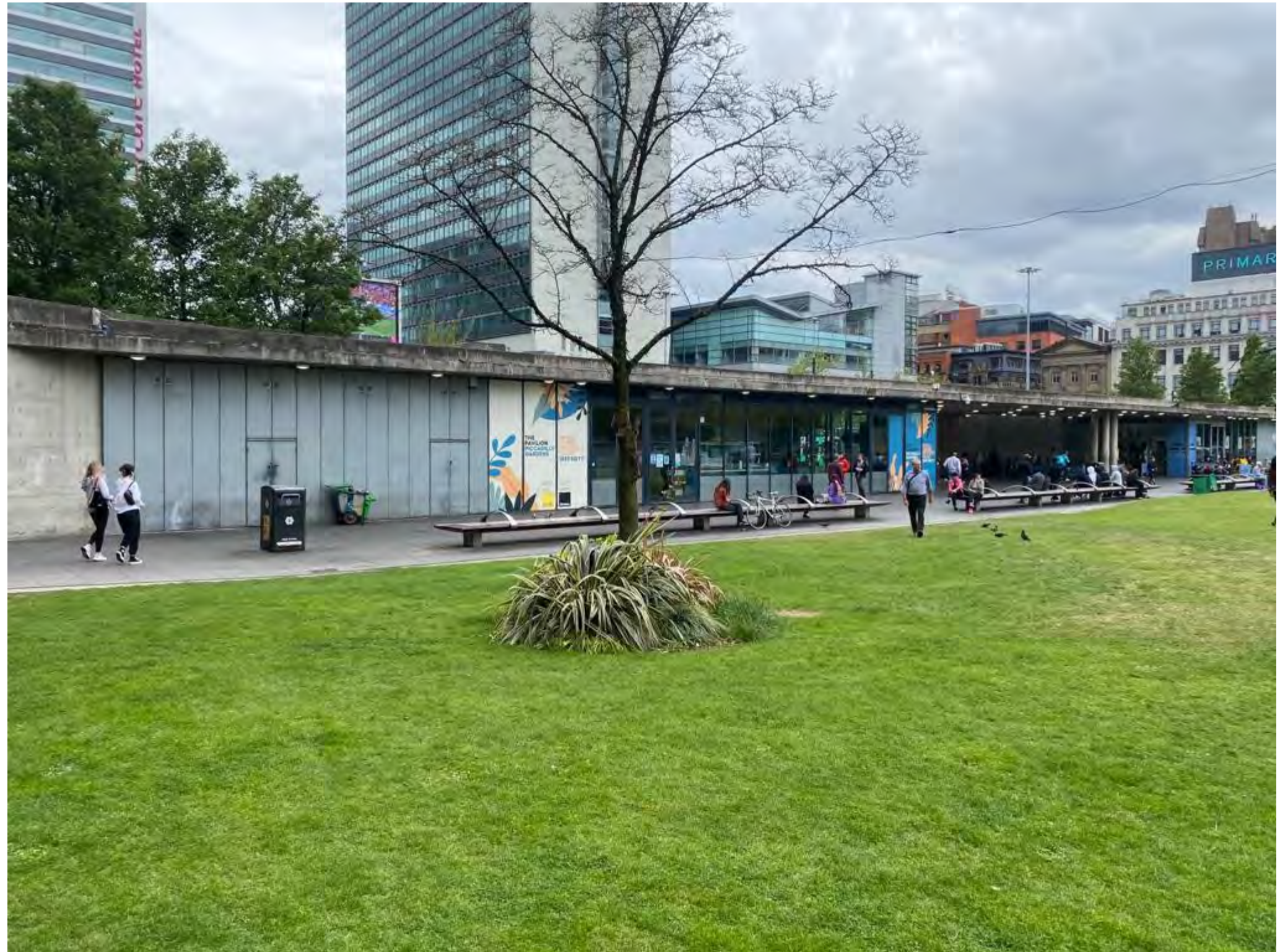
View looking at the shop front side of the Pavillion from Piccadilly Gardens
