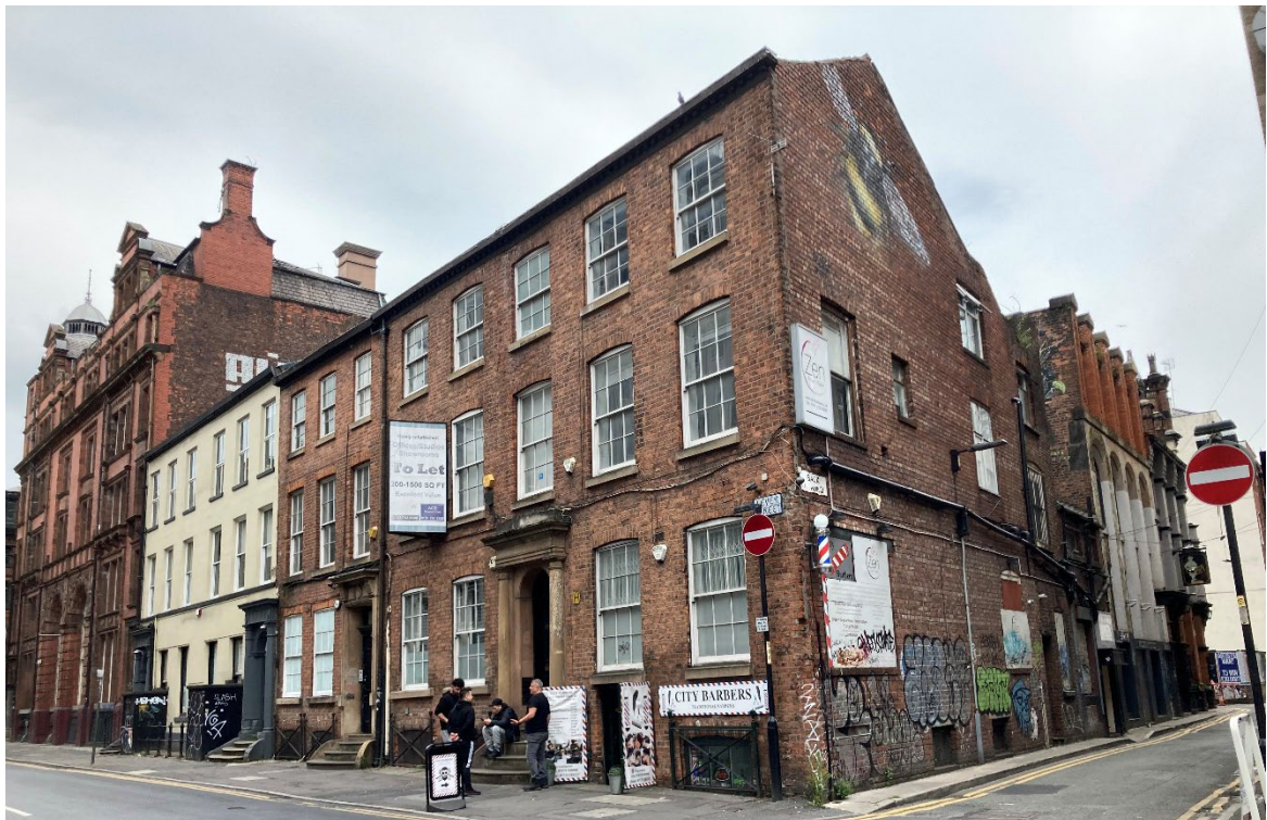
Photograph 11: Properties along Lever Street, characteristic of the surviving Victorian townscape
