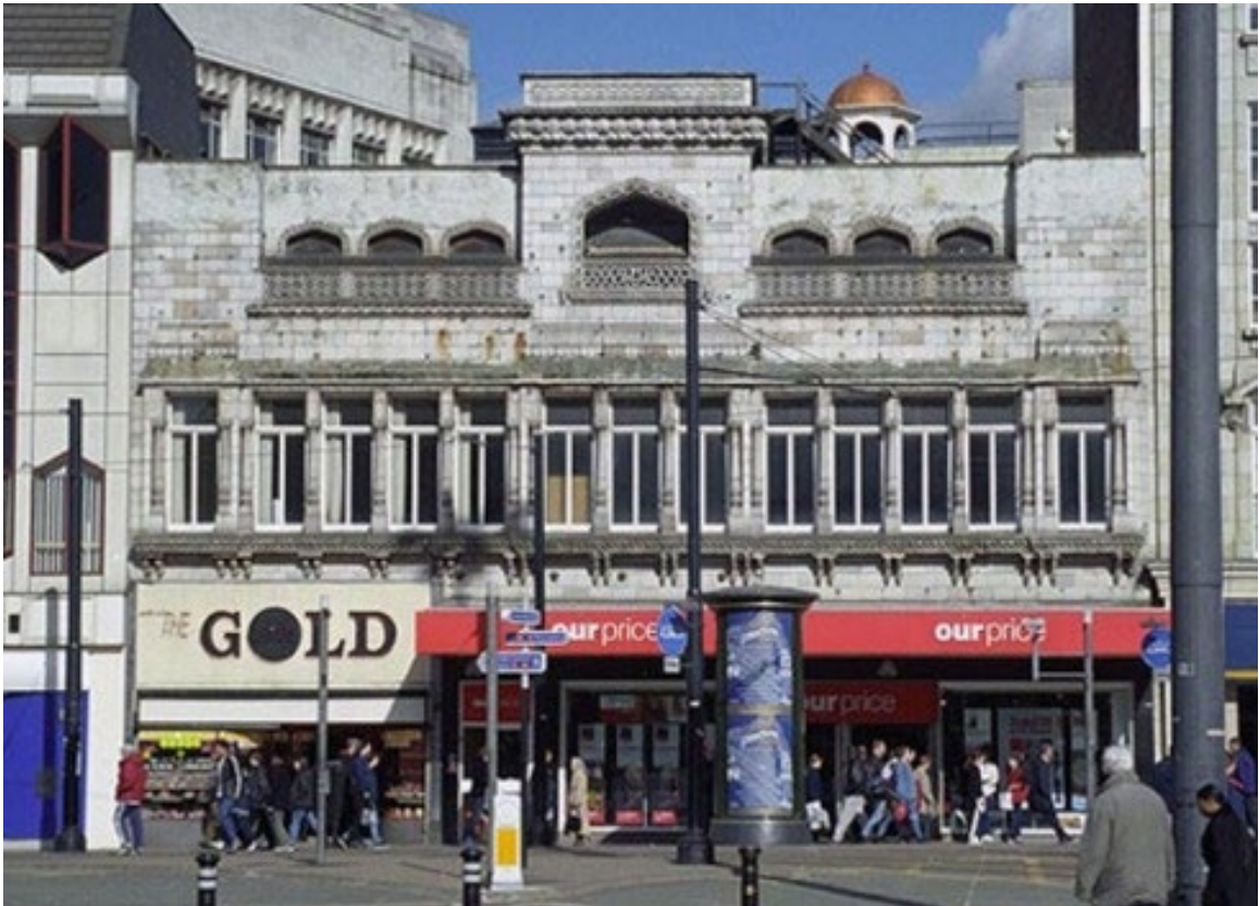
Photograph 4: Site, prior to demolition of the former Lyon's Cafe
