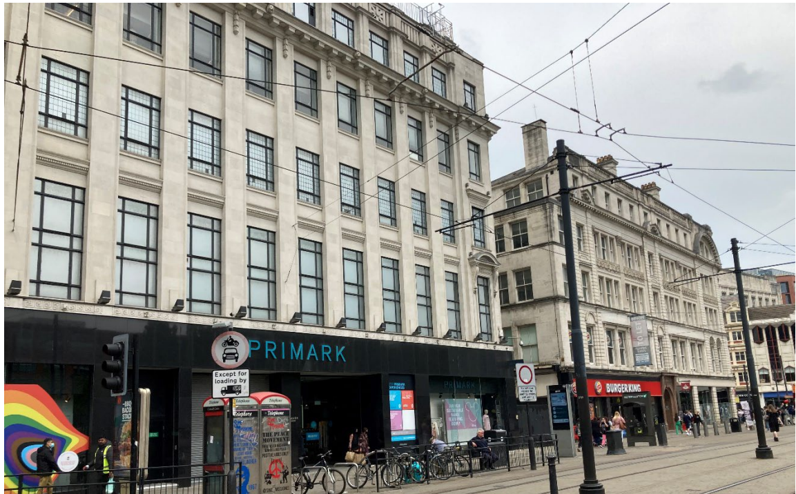
Photograph 8: View looking west along Market Street towards the southern boundary of the conservation area
