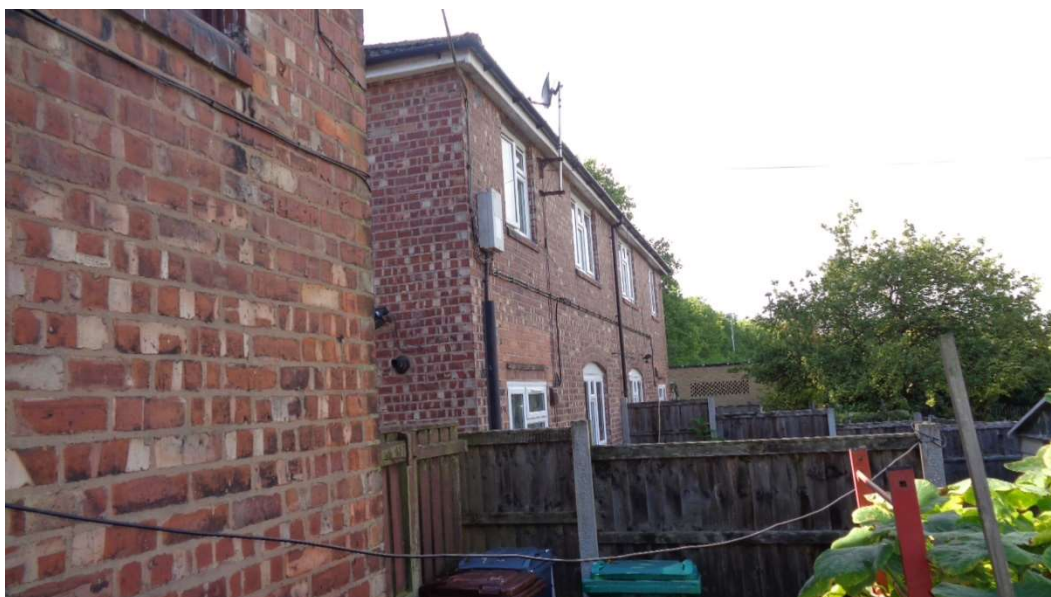
Adjacent Rear Property-82 Old Hall Lane
