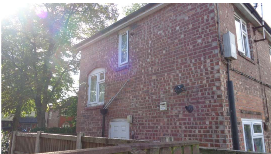
Gable of 80 Old Hall Lane facing adjacent property-78 Old Hall Lane
