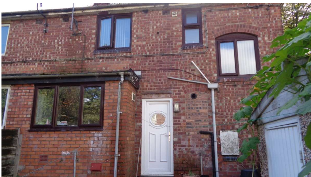
Rear Elevation of 80 Old Hall Lane
