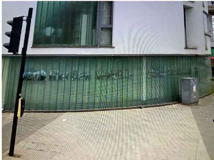
EXAMPLE OF BACK-LIT FROSTED GLAZING AT TRANSPORT HOUSE, CHAPEL STREET, SALFORD
