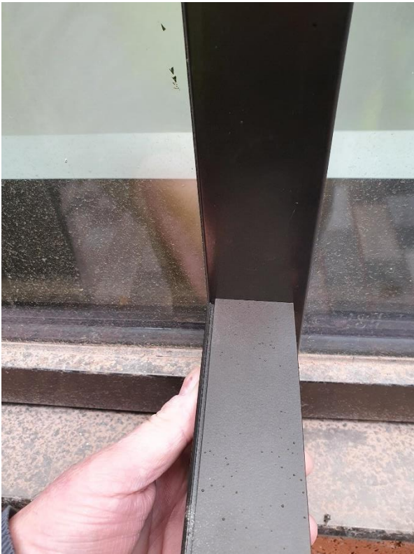
Double glazed aluminium window frame (bronze anodized)
