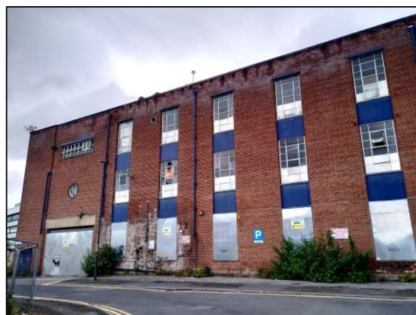
Photo 2: Eastern elevation, southern end
