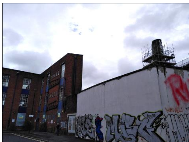
Photo 1: Eastern elevation, northern end
