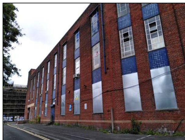
Photo 4: Western elevation, southern end
