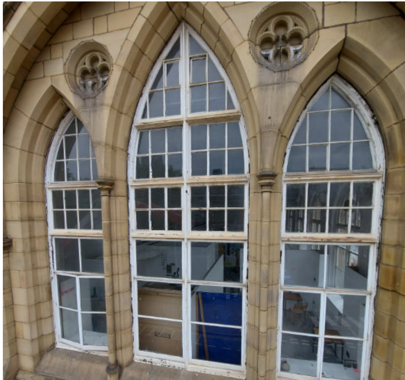
Cavendish Street - depressed tripartite stone arches
