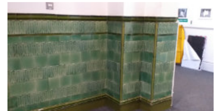
Wall tiling to Holden Gallery Foyer
