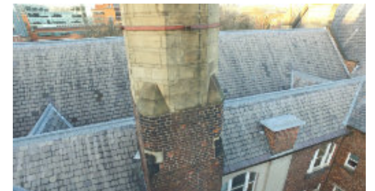
Internal roof courtyard - view towards North East
