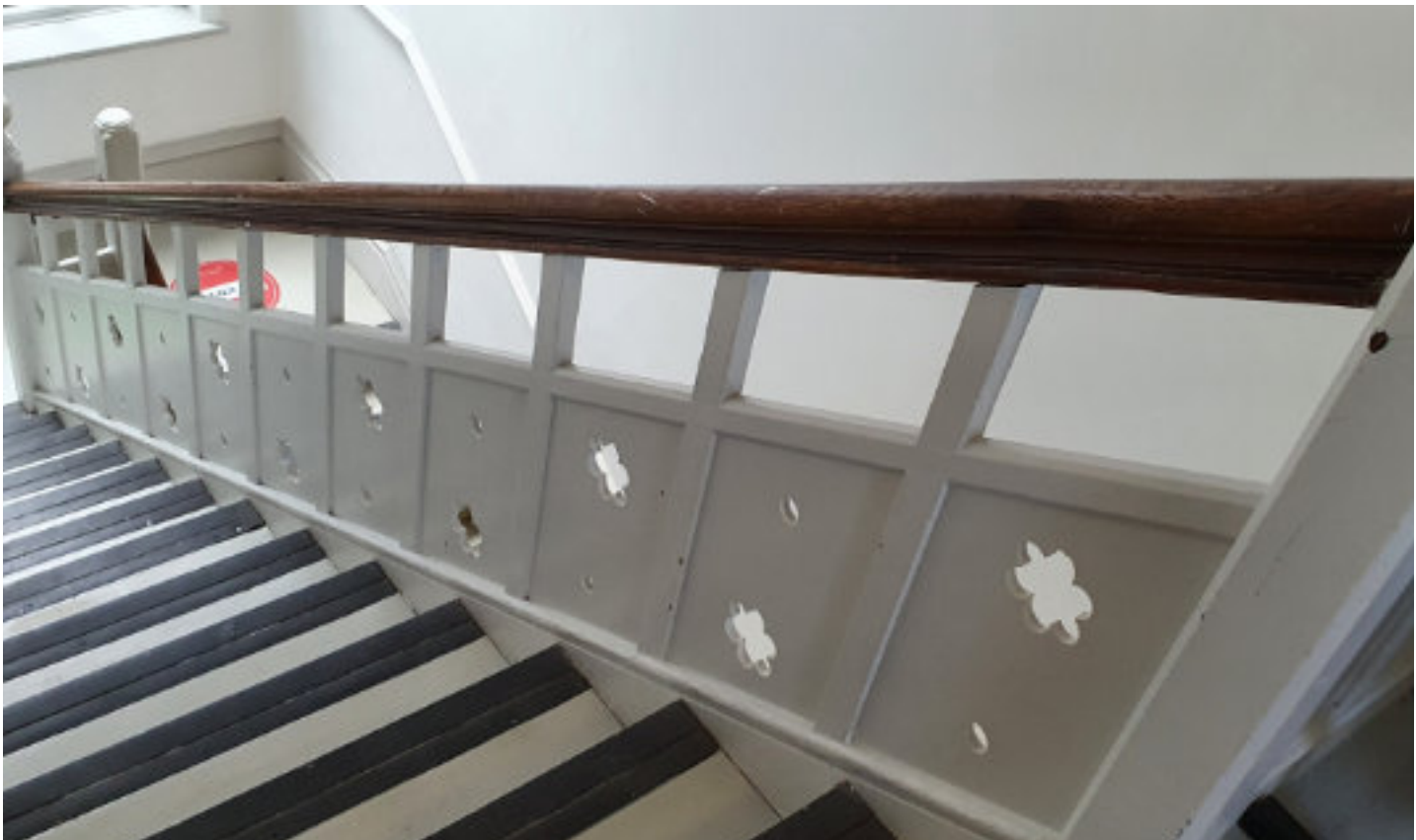
Stair 02: Existing Stair Handrail & Panelled Baluster - Asset of Significance
