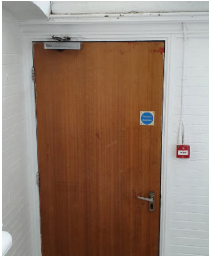
Category 2: Existing modern door of poor quality
