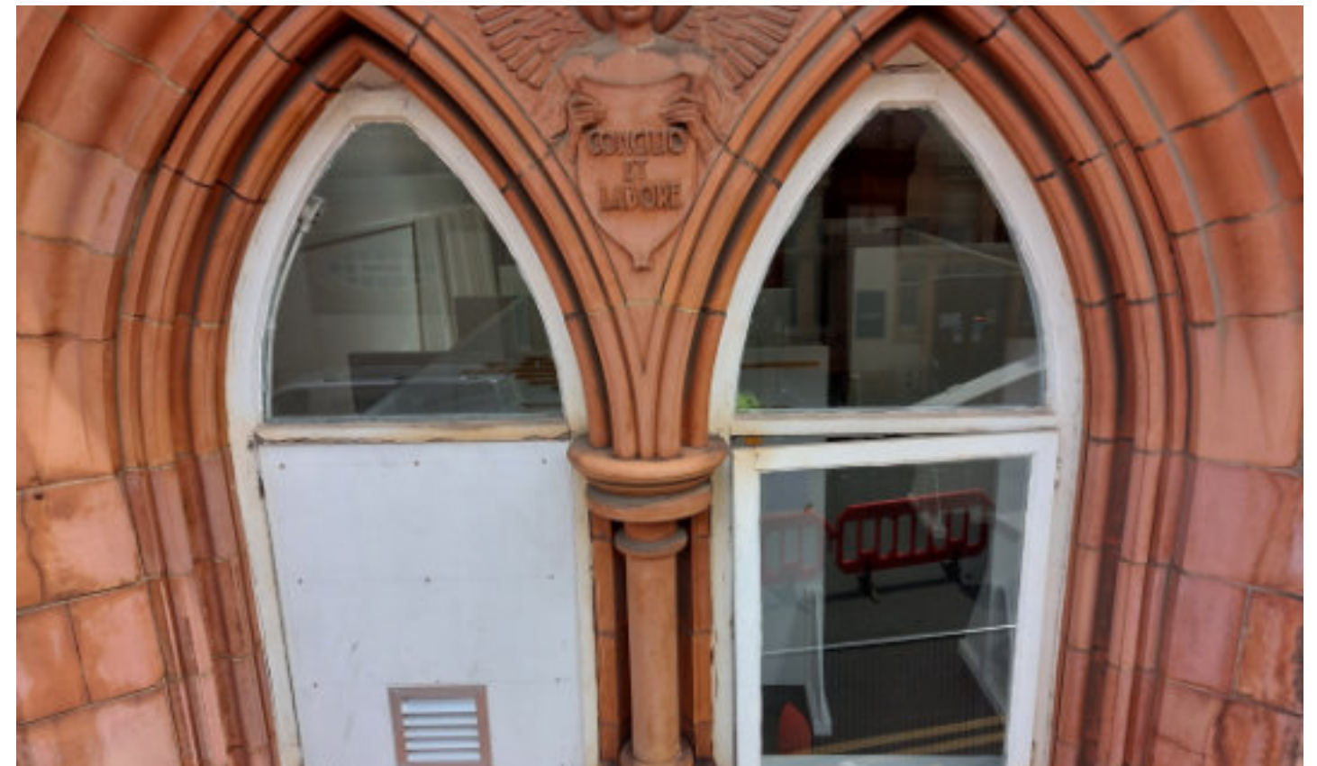
Non original timber frame and service spandrel panels / clear glazing
