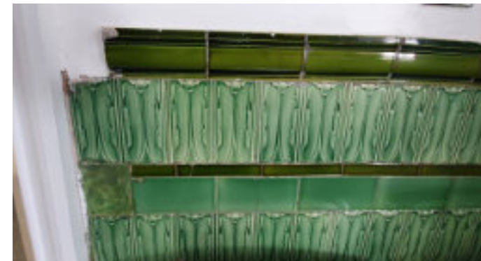
Wall tiling to Holden Gallery Foyer
