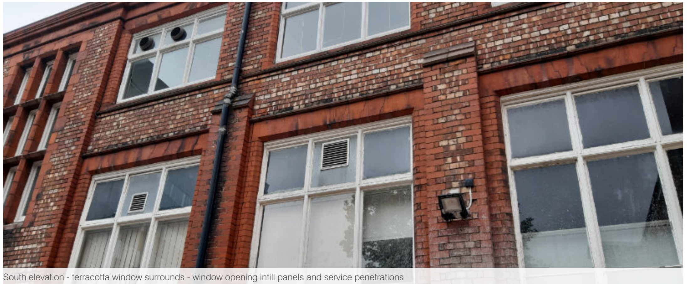
Typical window condition - terracotta pilaster
