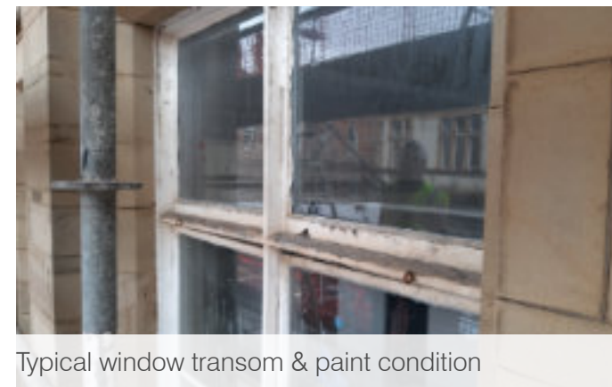
Typical window transom & paint condition
