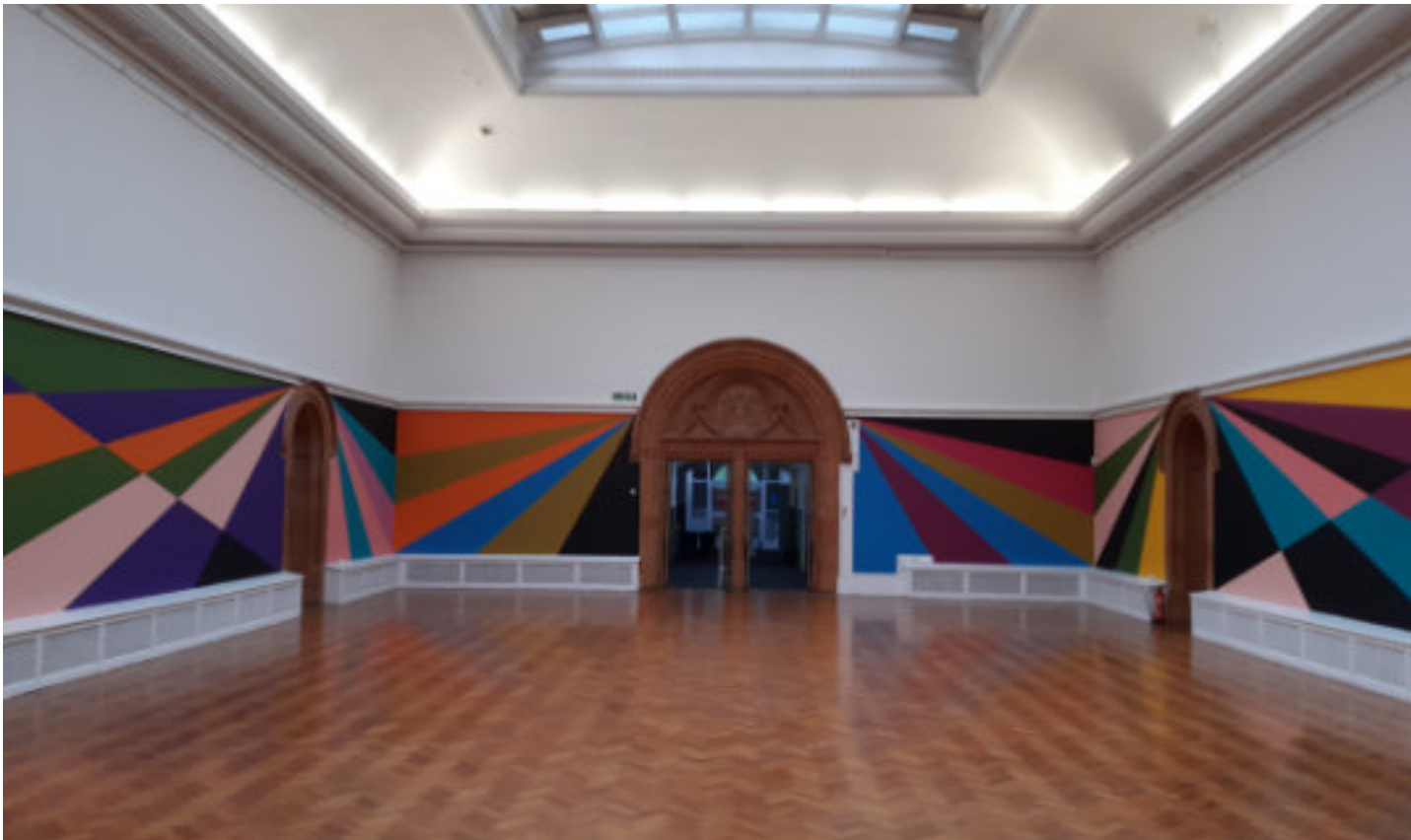
Holden Gallery & Existing Timber block varnished parquet flooring
