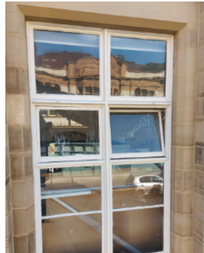
Timber in general good condition - mix of glazing
