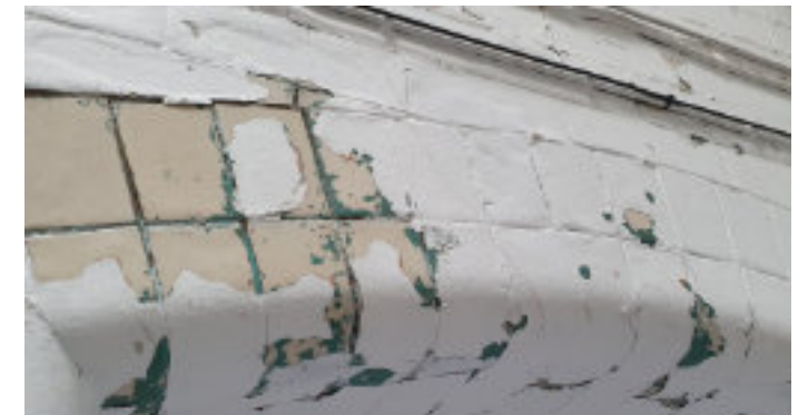
Existing Glazed Bricks to Staircase 01 & 05
