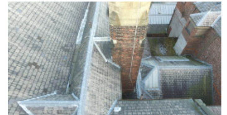
Internal roof courtyard - view towards Ginnel
