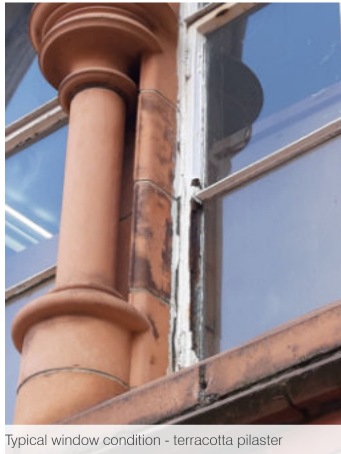
Typical window transom & paint condition
