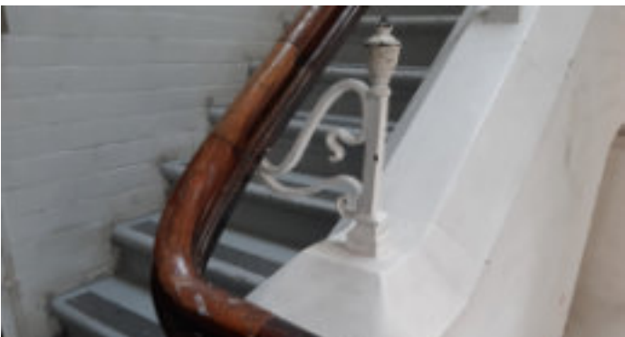
Stair 01: Existing Stair & Handrail - Asset of Significance
