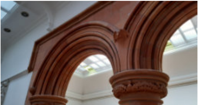
Terracotta columns within the Holden Gallery
