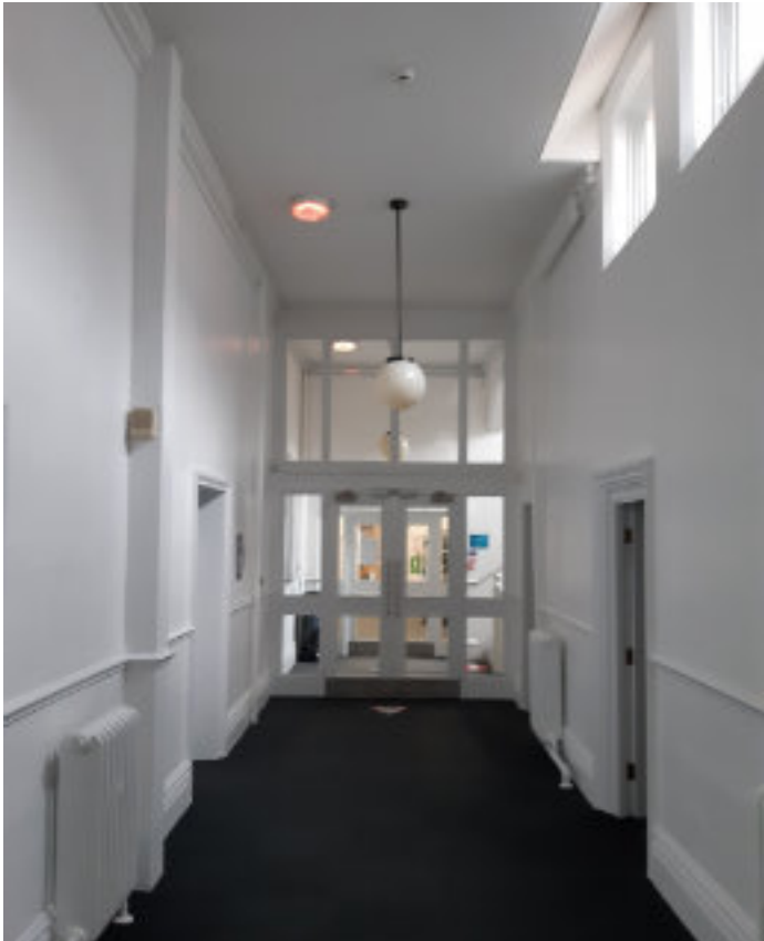
Existing ground floor corridor and carpet finish
