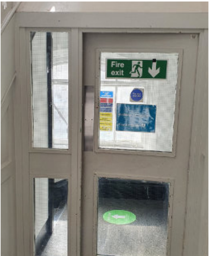
Category 2: Existing modern door of poor quality
