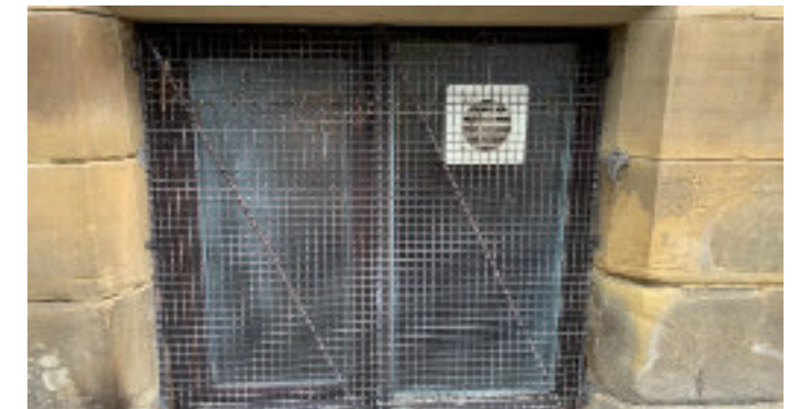
Modern frame with services + security mesh - replace
