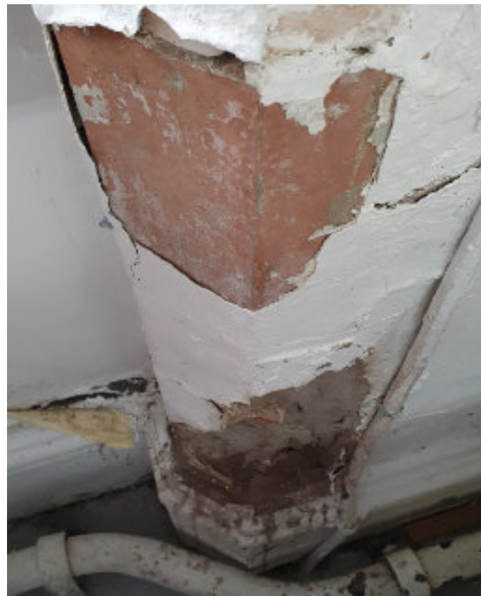
Terracotta Window Surround to First Floor corridor
