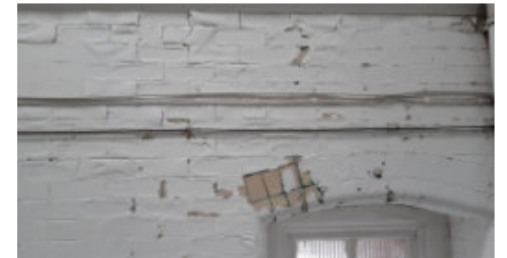
Existing Glazed Bricks to Staircase 01 & 05
