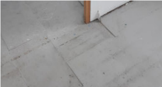
Existing painted timber floor
