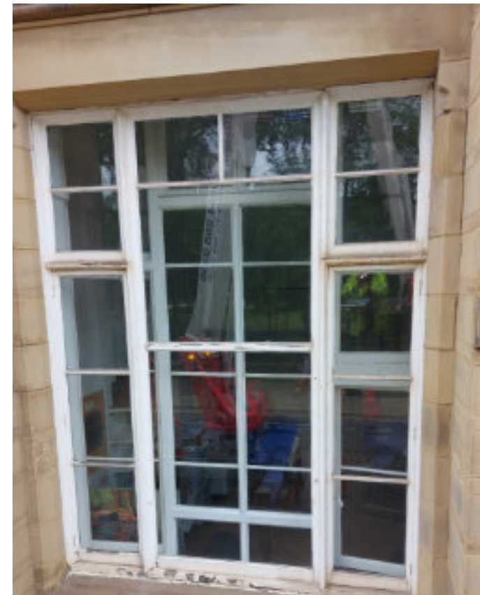
Outer frame altered from original - to be restored
