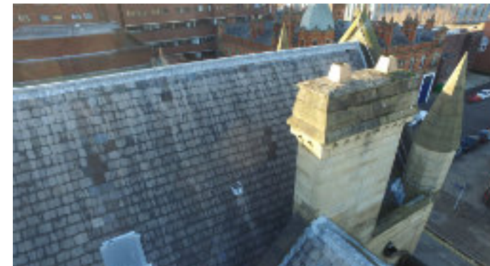
Perimeter roof - view towards North West
