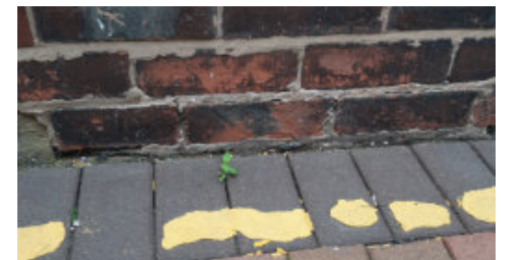
Raised external levels
