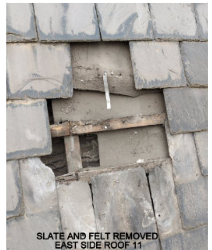
Typical roof build up to Roof 11
