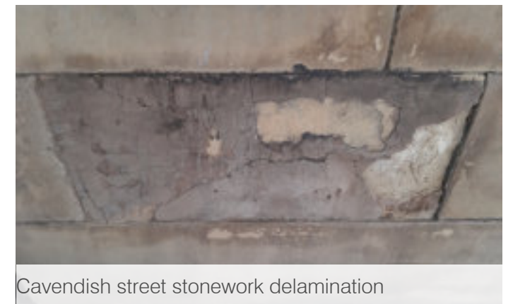
Cavendish stonework delamination
