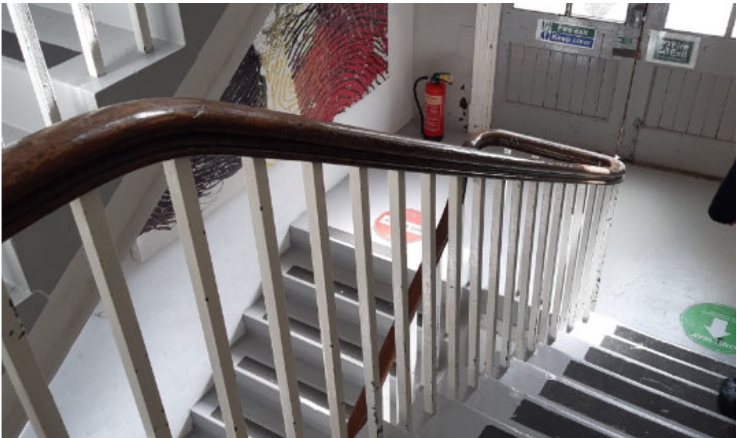
Stair 05: Existing Stair Handrail - Asset of Significance
