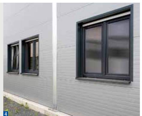
3-4 Double-wing tilt and turn windows in a gable wall with insulated panels. Integrated into the warehouse is an office block with more than 400 m 2 including an entrance area consisting of a three-bladed glass door and a steel awning.
