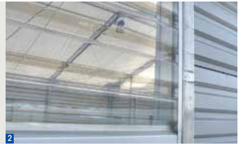
1-2 Transparent plastic panels are a cost-effective and easy to assemble solution to supply additional light to trapezoidal sheet metal structures.
