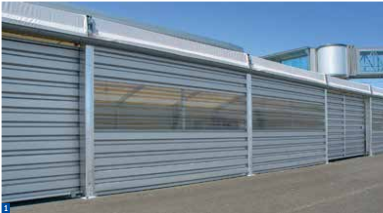
1-2 Transparent plastic panels are a cost-effective and easy to assemble solution to supply additional light to trapezoidal sheet metal structures.
