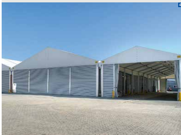
2-5 The translucent roof tarpaulins create excellent light conditions ideal for warehousing applications 24/7.
