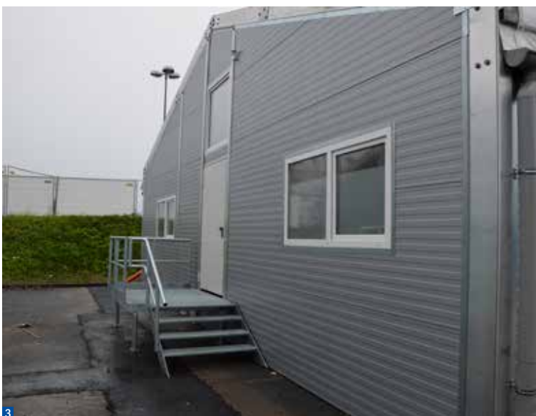
3-4 Double-wing tilt and turn windows in a gable wall with insulated panels. Integrated into the warehouse is an office block with more than 400 m 2 including an entrance area consisting of a three-bladed glass door and a steel awning.
