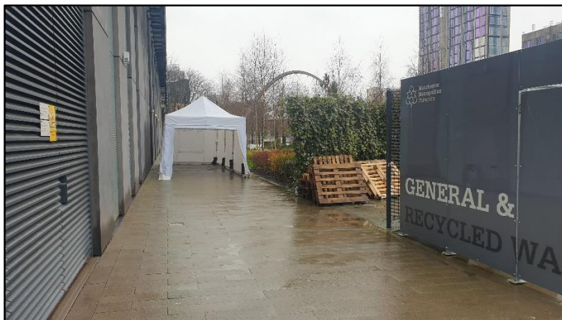
Figure 3: Hardstanding areas on site
