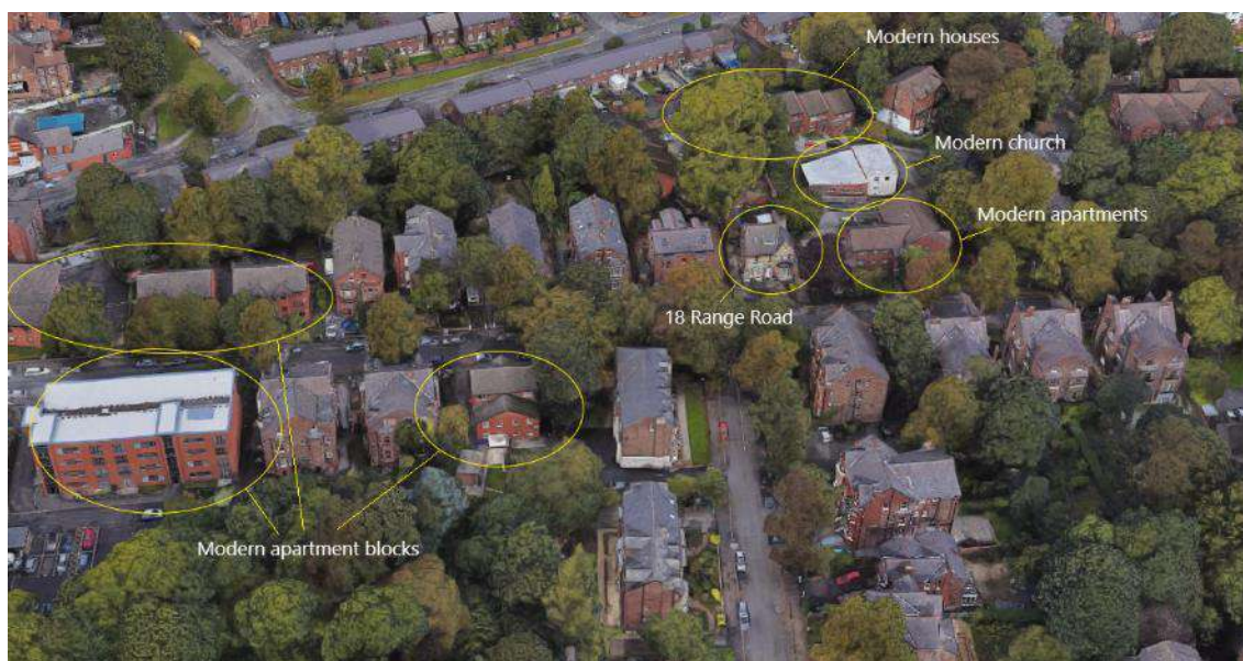
Figure 8) Aerial view showing later C20th development in the vicinity of 18 Range Road
