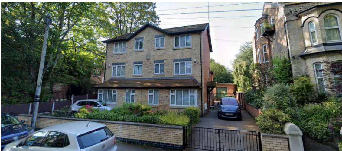
Figure 7) Modern housing on south side of Range Road
