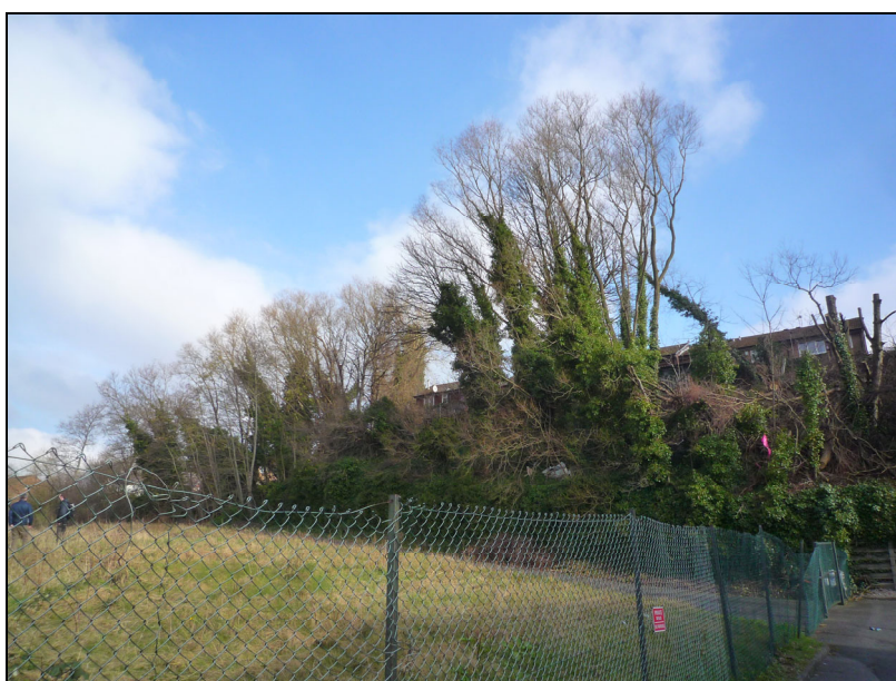
P2 – G5 & G6 viewed from east
