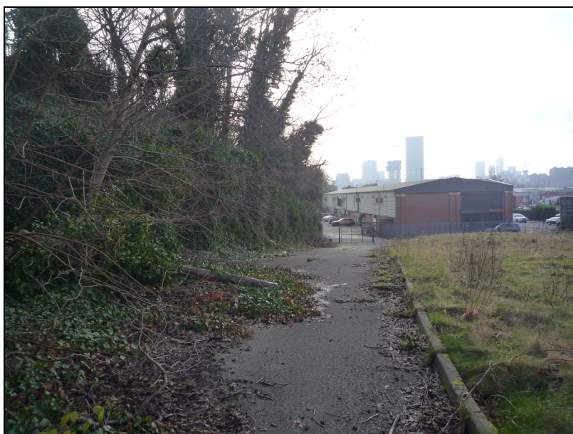
P3 – Existing retaining wall to south of G6
