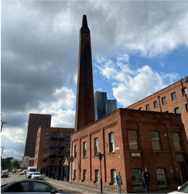
Figure 4.3 - Listed Building 2: Mill Chimney Stack, from Hulme Street looking north (Authors own, 2021)
