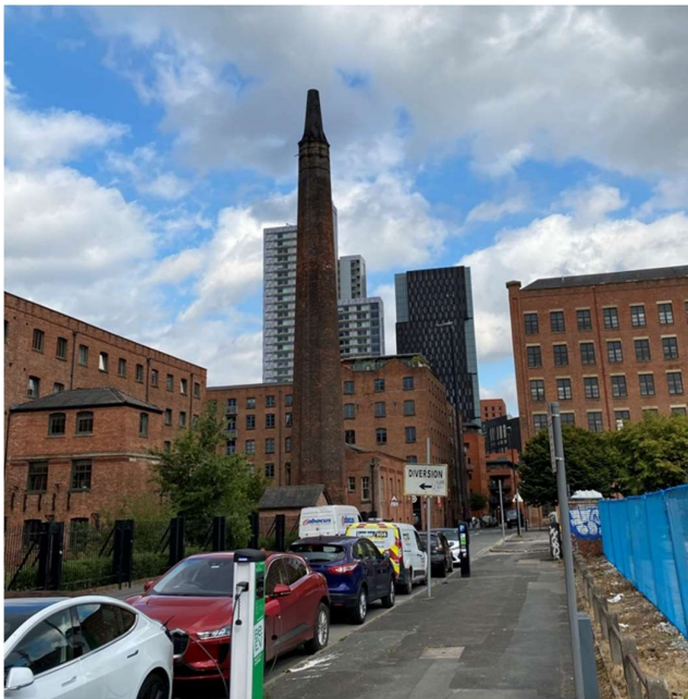
Figure 5.2 - Mill Chimney Stack
