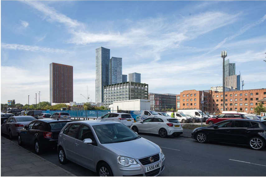
Figure 6.6: View 3: Looking north from the junction of Cambridge and Chester St, including Proposed Development
