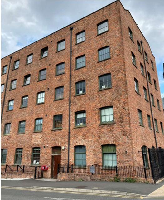
Figure 4.2 – Listed Building 1: Former Cotton Mill, looking east (Author's own, 2021)
