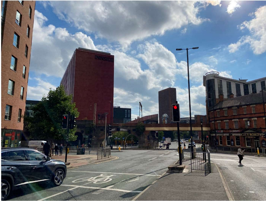
Figure 4.8 – Listed Asset 6: Listed Viaduct taken from Whitworth Street West facing south towards the site (Author's Own 2021)
