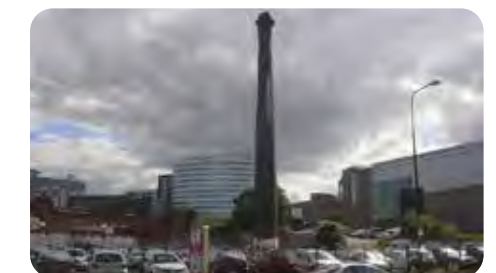
Chimney before demolition, 2007
