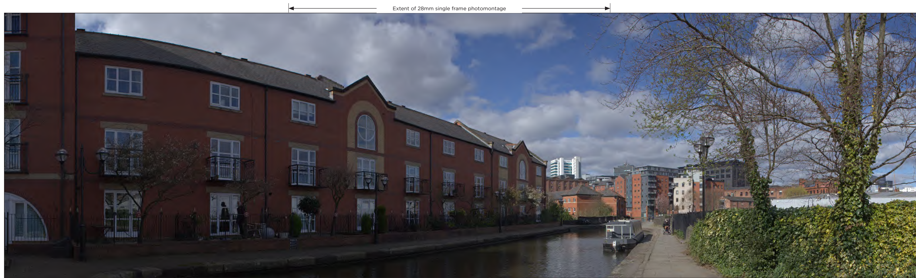
Grid Reference: 385081E 398108N Horizontal Field of View: 90°
