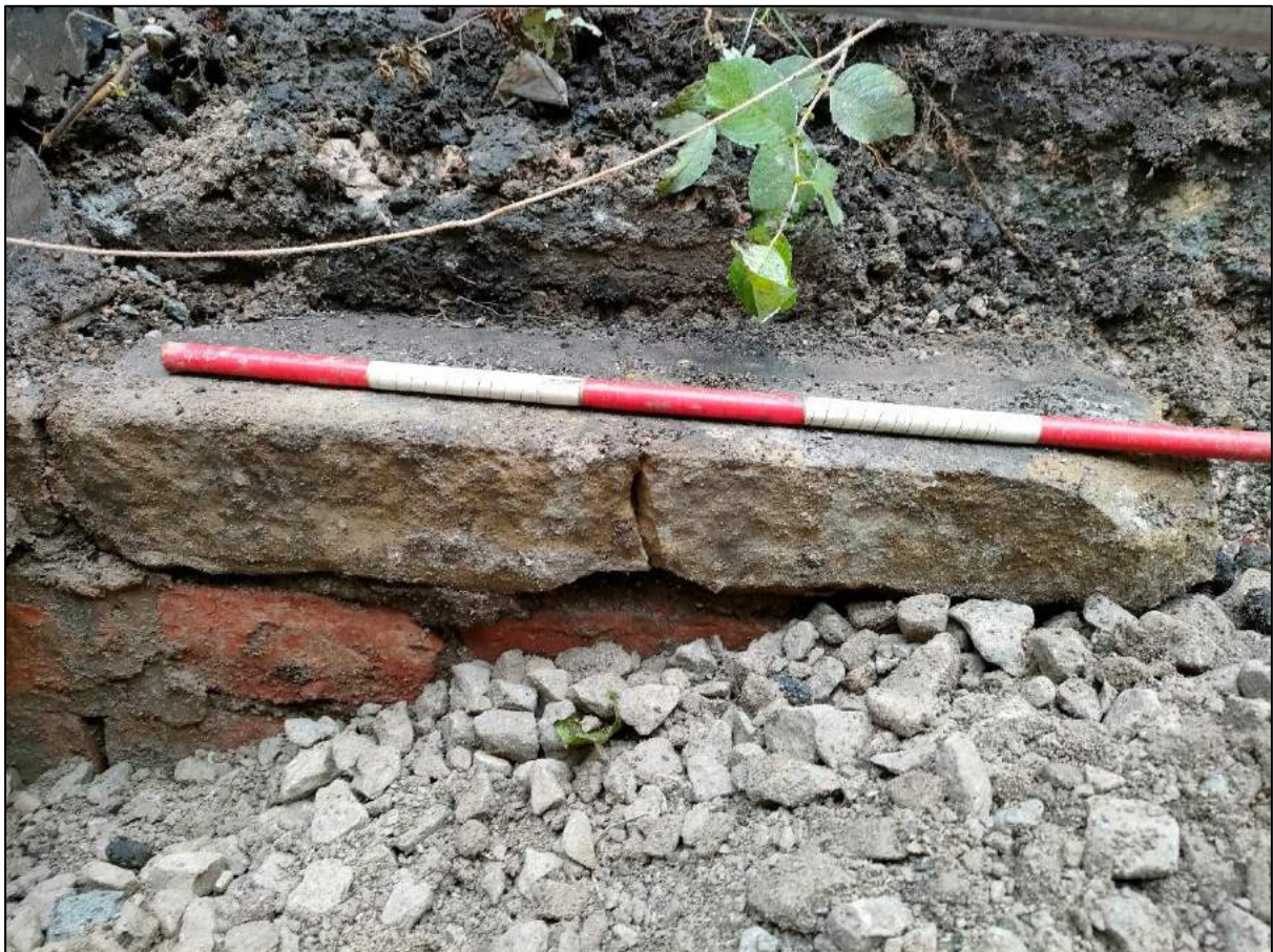
Northern side of large drain next to carpark wall showing sandstone caps
