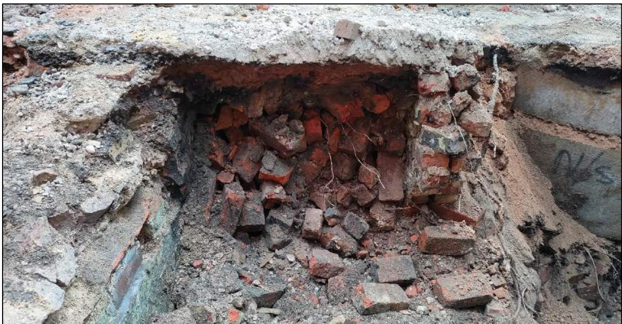
Dividing wall at S end of cellars looking W.
