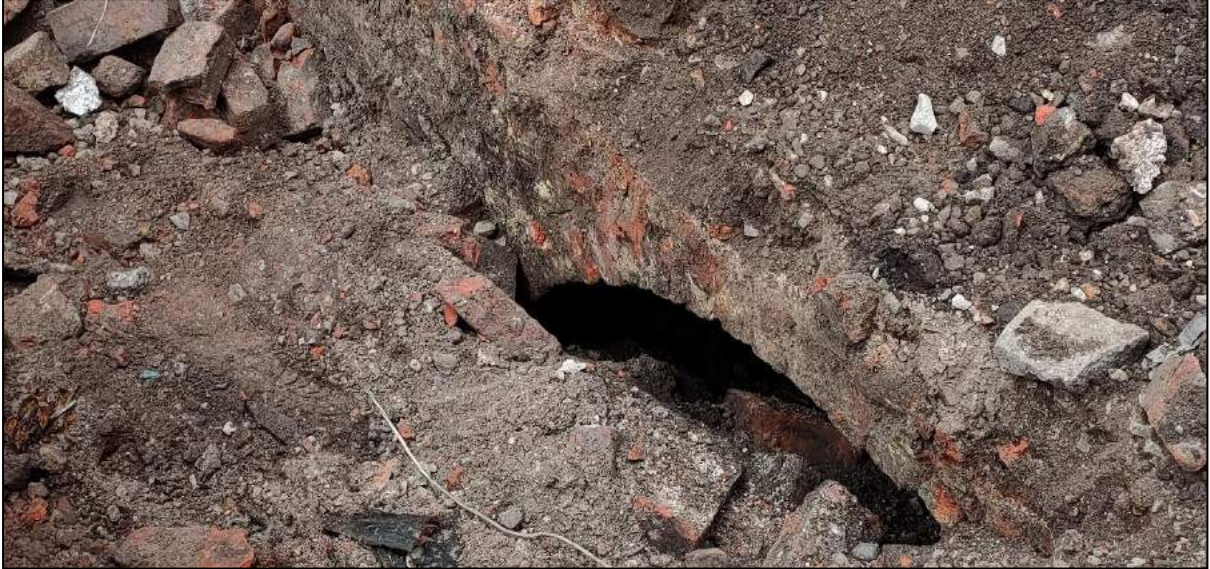
Cellar vault roof looking NE
