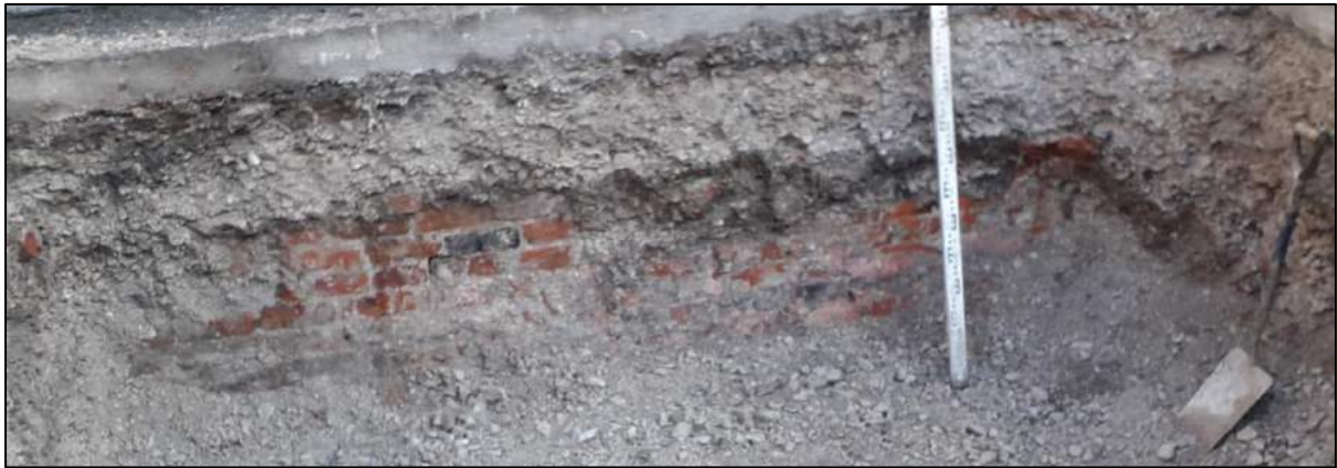
Wall in Planter 4 looking N
