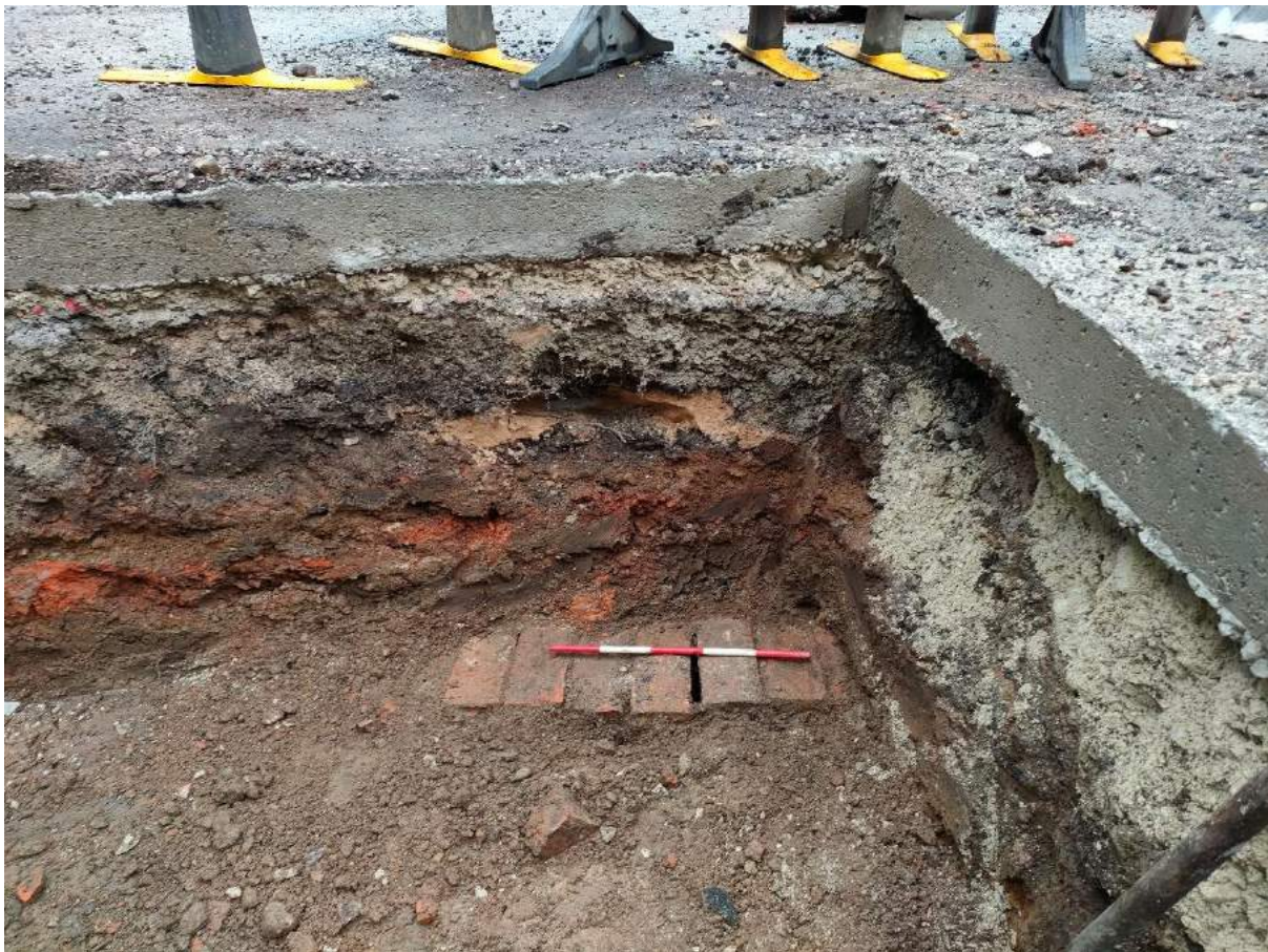
Drain channel prior to lifting the caps.
