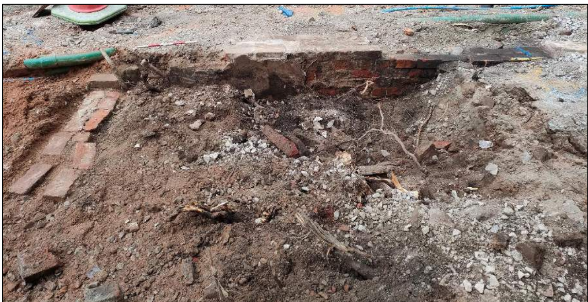
E-W wall with render, dividing wall and plumbing
