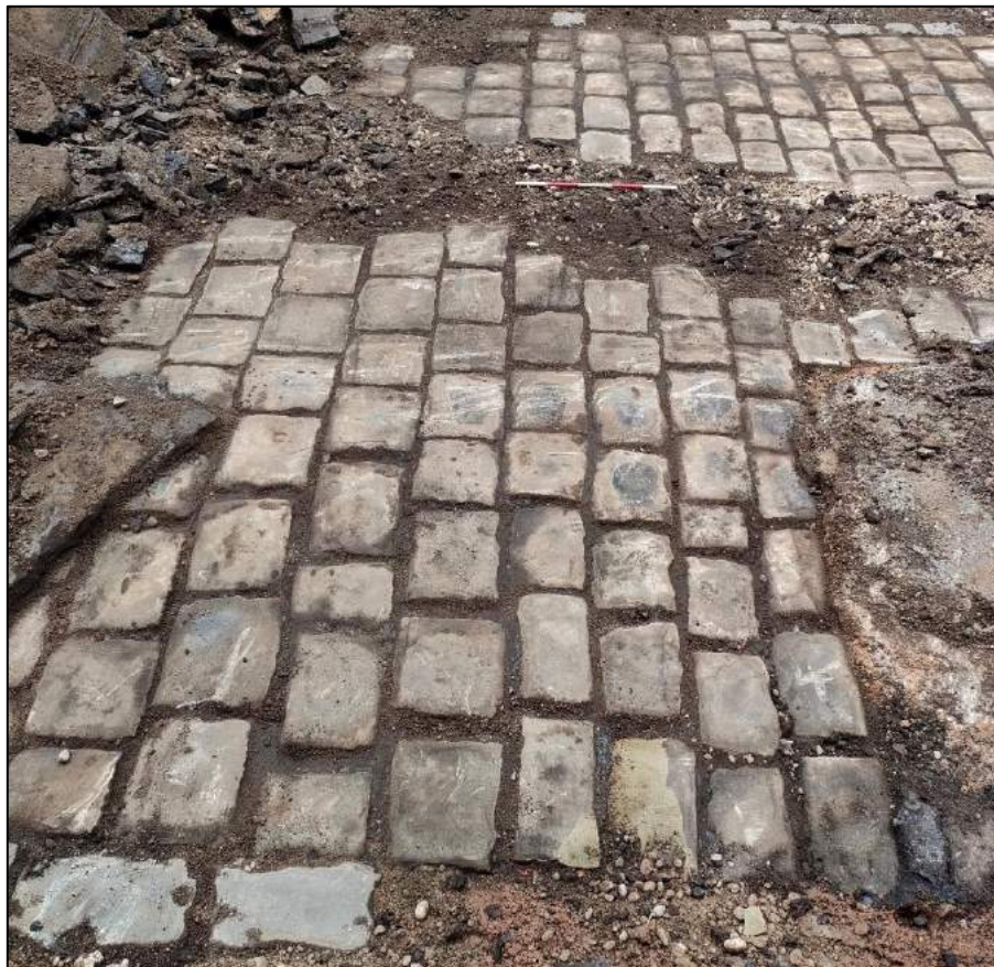
Flattened setts in the centre of the road and rounded ones at the sides
