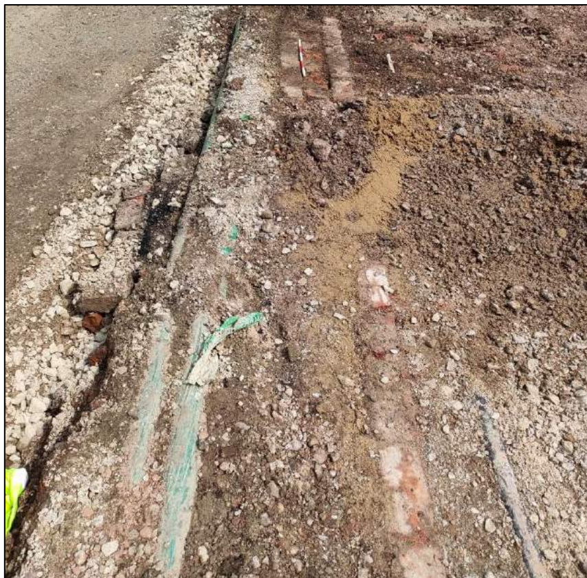
E-W wall, possible coal chute on left of green Virgin conduits
