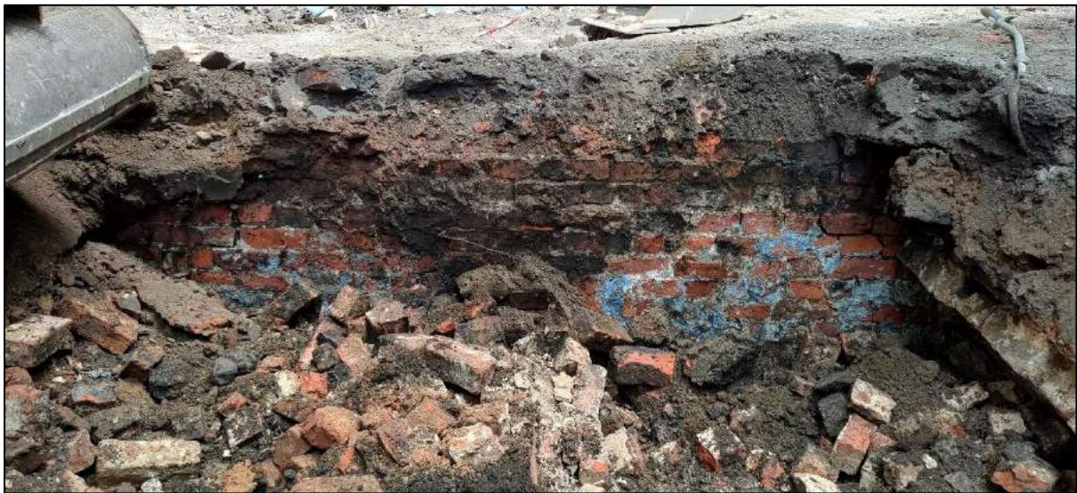
Dividing wall between the two arches removed.
