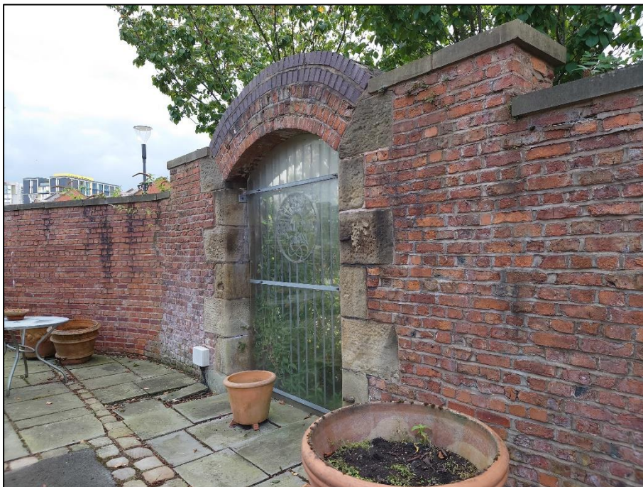
Photograph 3 showing part of the wall
