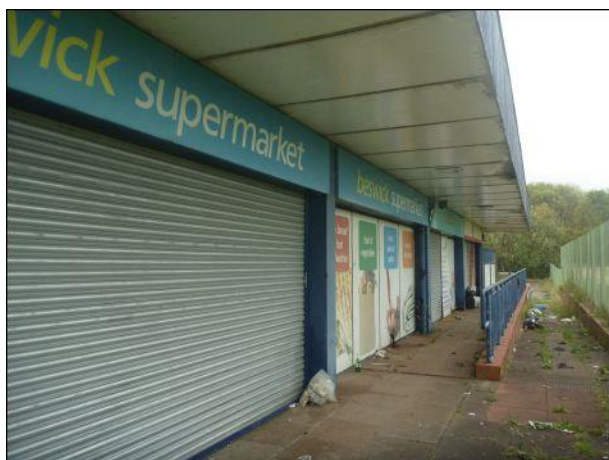
Photo 9: Building 1, south-western elevation, northern end
