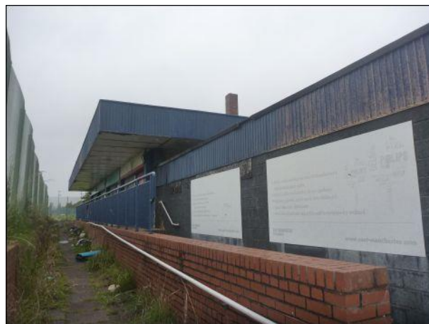
Photo 8: Building 1, south-western elevation, southern end
