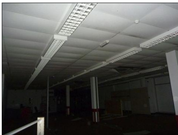
Photo 15: Building 1, former supermarket
