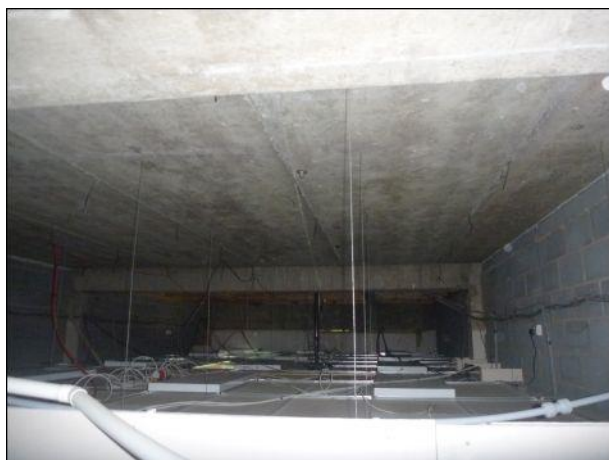
Photo 17: Building 1, void above former supermarket
