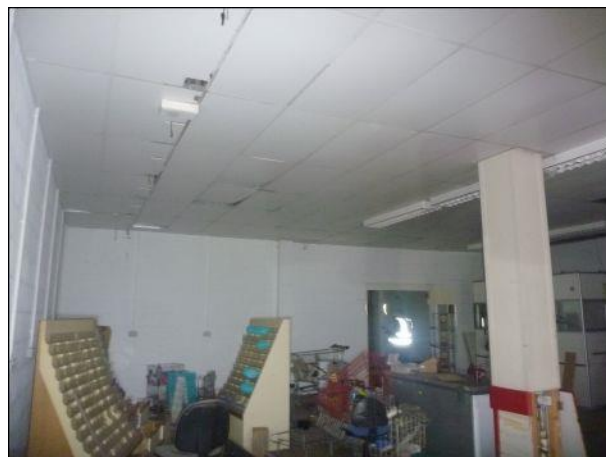
Photo 14: Building 1, former supermarket
