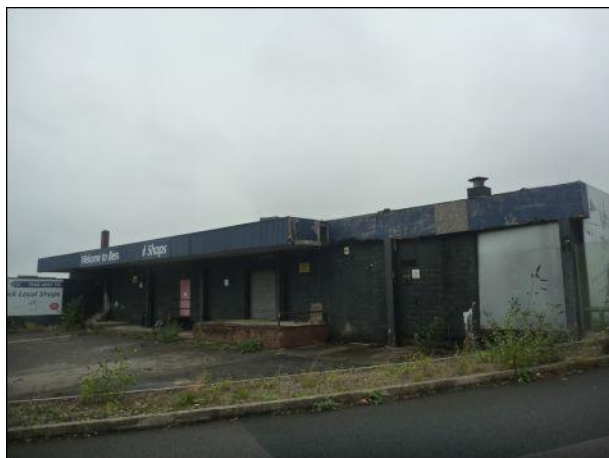
Photo 7: Building 1, south-eastern elevation
