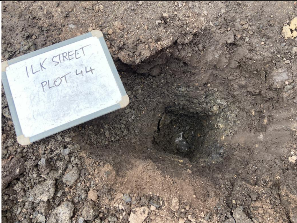
Photograph 3: Validation of Geotextile Membrane
