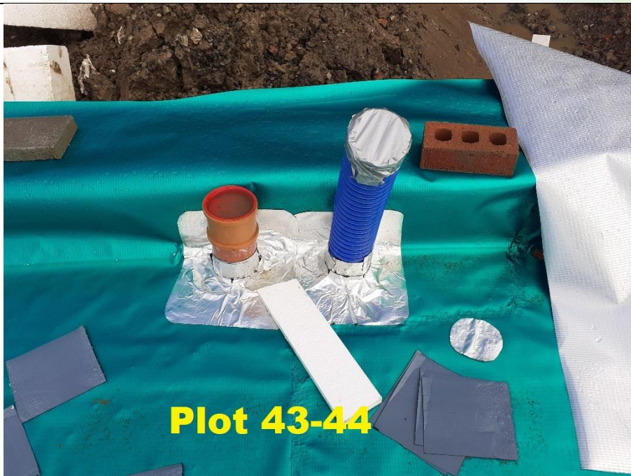
Photograph 8: Validation of Gas Membrane Installation (Please note, plots 43 and 44 are semidetached and were validated together. Gas membranes are satisfactory within both plots)
