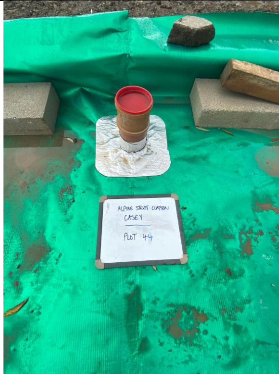
Photograph 7: Validation of Gas Membrane Installation
