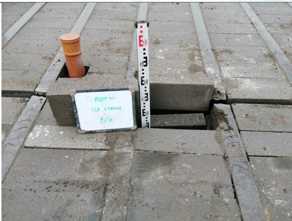
Photograph 4: Validation of Sub-Floor Void Space (min 150 mm)
