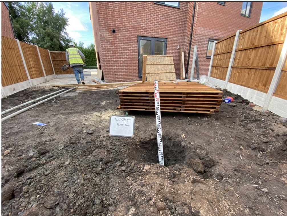
Photograph 2: Validation of Garden Capping Thickness
