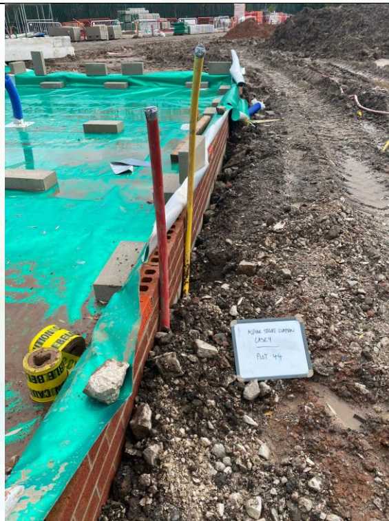
Photograph 6: Validation of Gas Membrane Installation
