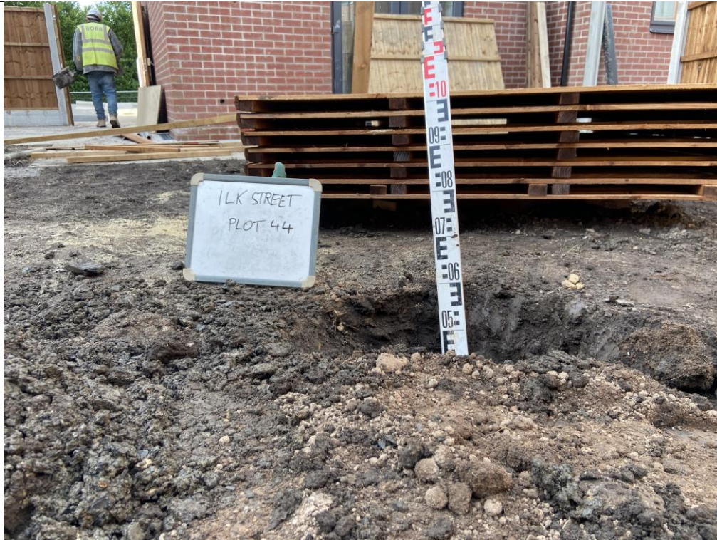
Photograph 1: Validation of Garden Capping Thickness
