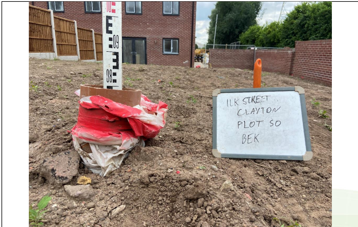
Photograph 1: Validation of Garden Capping Thickness (Plot 51, not 50)
