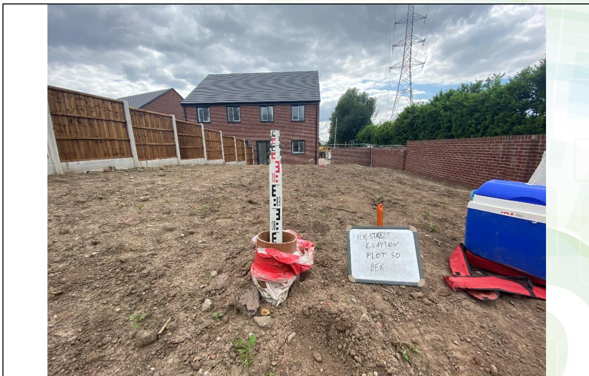
Photograph 2: Validation of Garden Capping Thickness (Plot 51, not 50)
