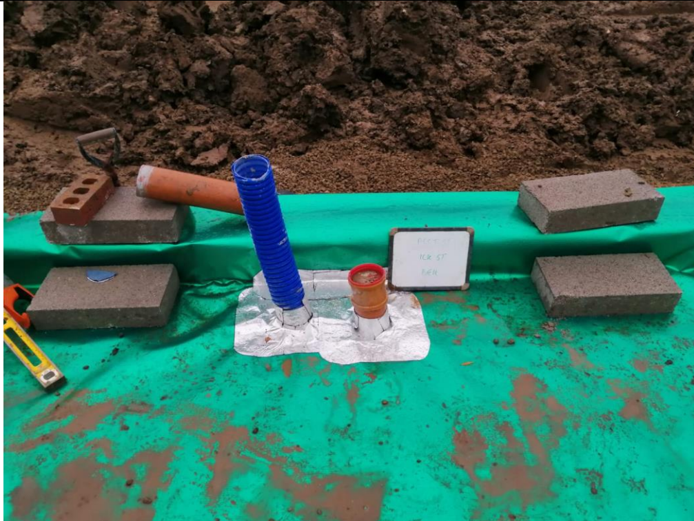
Photograph 7: Validation of Gas Membrane Installation
