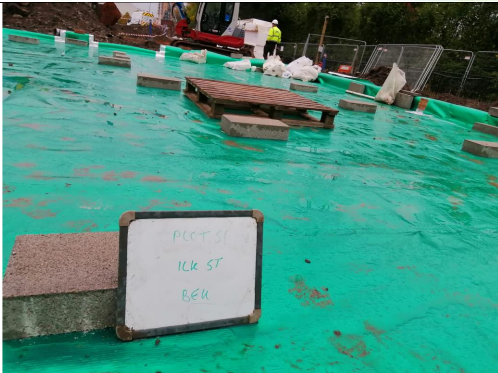
Photograph 8: Validation of Gas Membrane Installation
