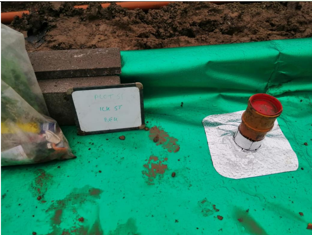
Photograph 6: Validation of Gas Membrane Installation
