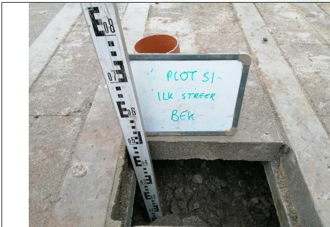
Photograph 4: Validation of Sub-Floor Void Space (min 150 mm)
