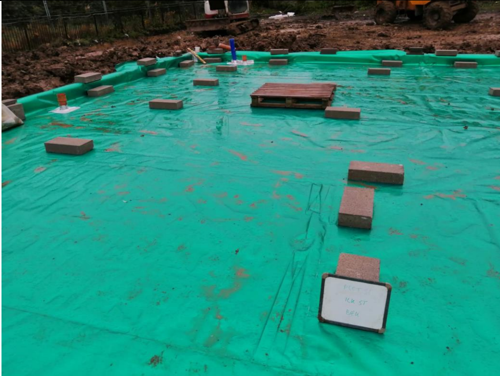
Photograph 5: Validation of Gas Membrane Installation
