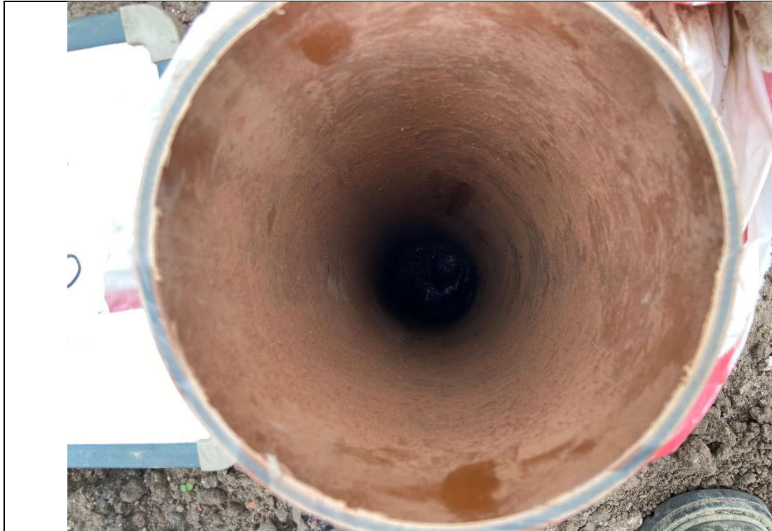
Photograph 3: Validation of Geotextile Membrane
