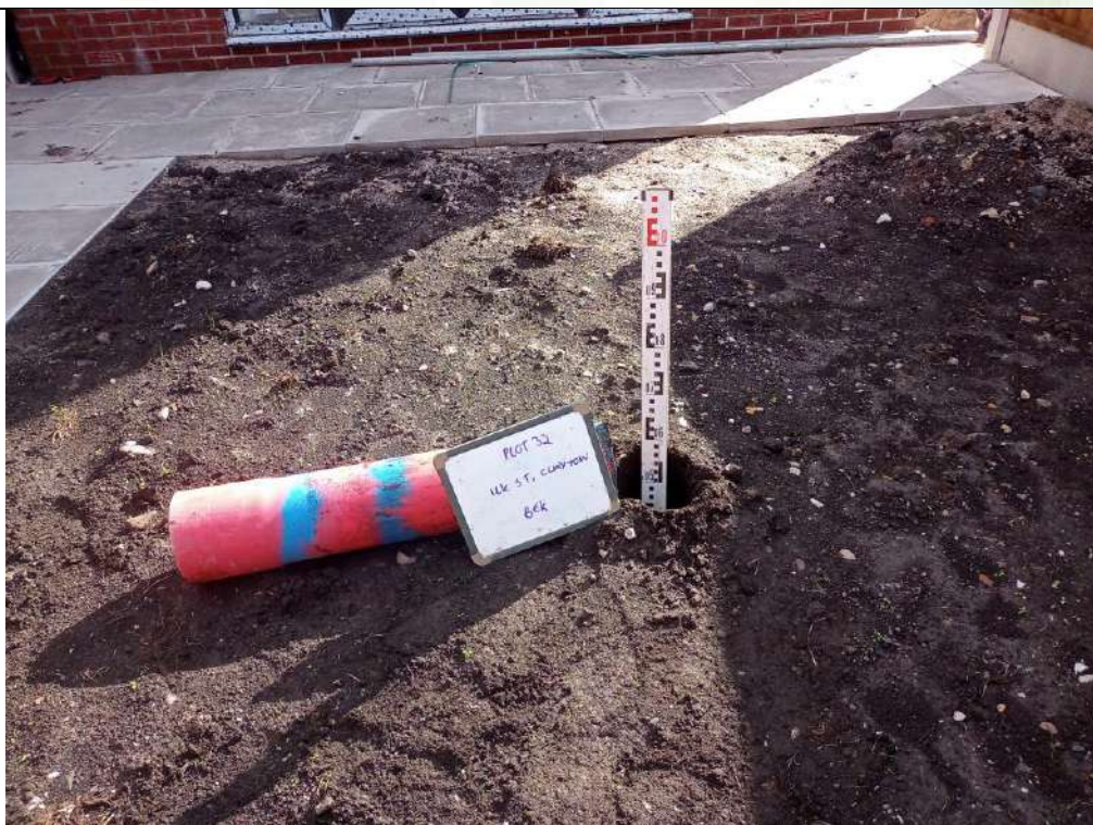
Photograph 2: Validation of Garden Capping Thickness
