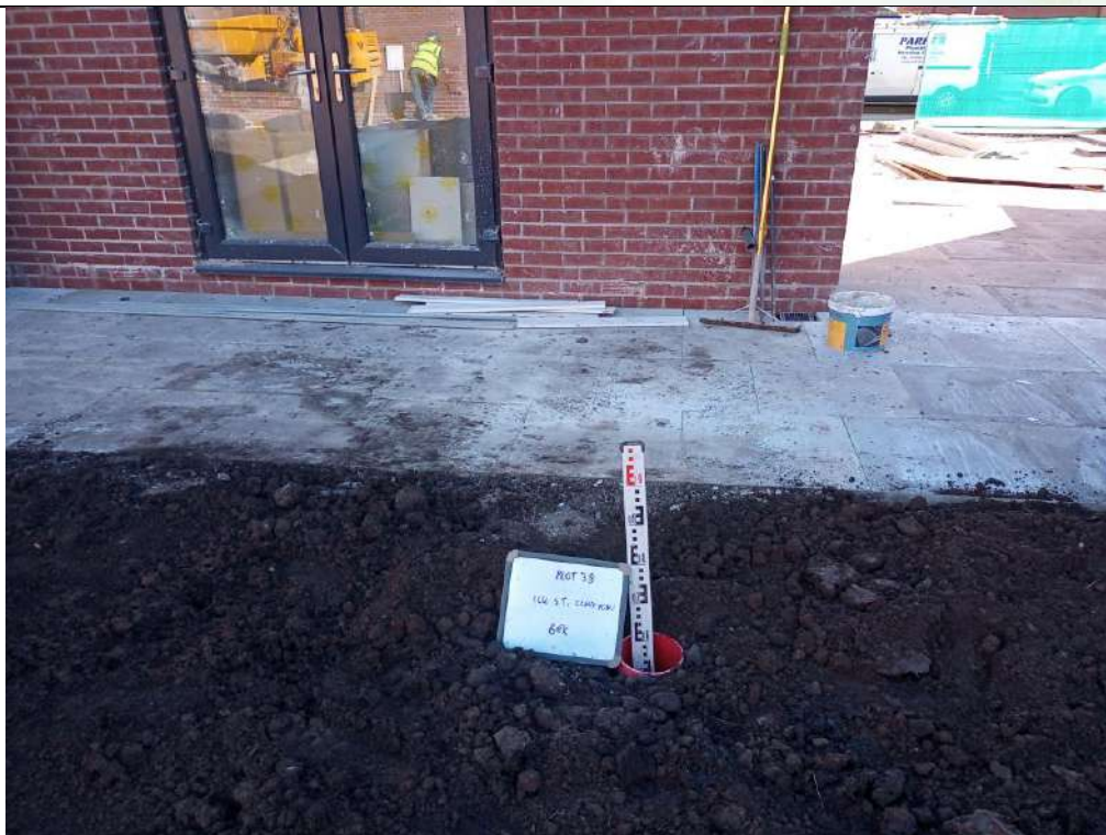
Photograph 2: Validation of Garden Capping Thickness
