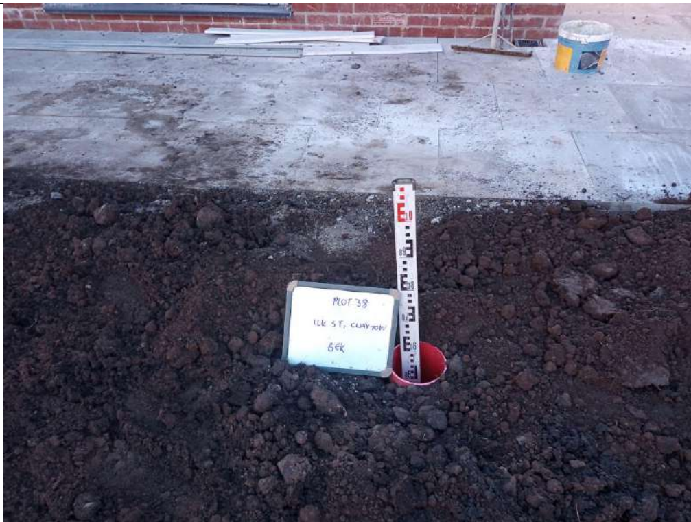
Photograph 1: Validation of Garden Capping Thickness
