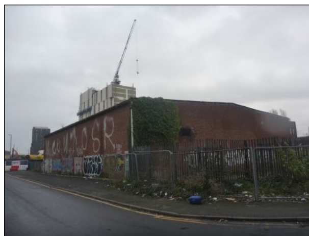
Photo 10: Building 10, south-western and north-western elevation
