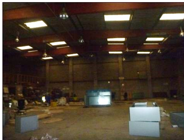
Photo 14: Building 10, internal area
