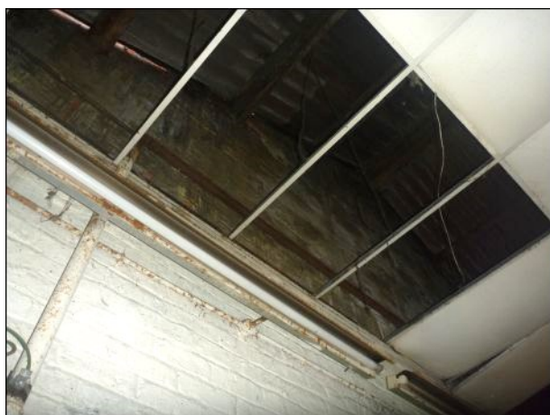
Photo 5: Building 2, north-eastern gable end
