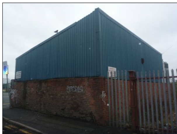
Photo 6: Building 3, north-eastern and north-western elevations
