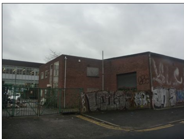
Photo 11: Building 10, north-eastern elevation
