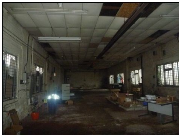
Photo 4: Building 2, internal area
