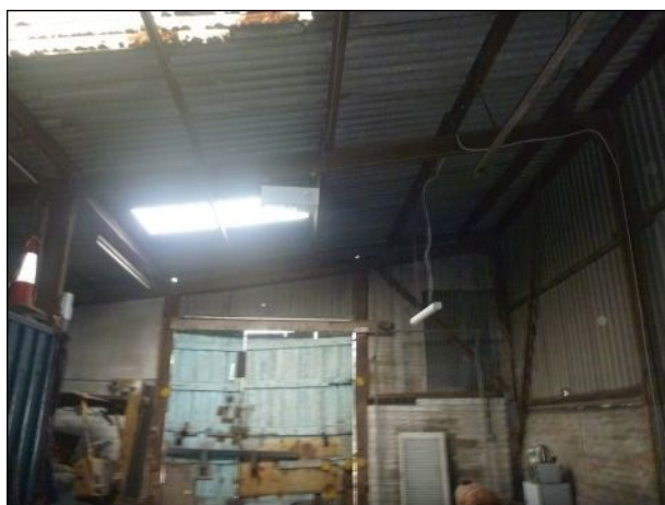
Photo 9: Building 3, internal area
