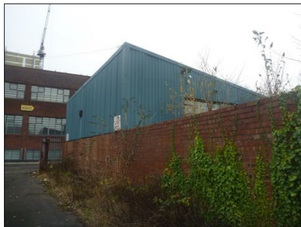
Photo 8: Building 3, north-western elevation
