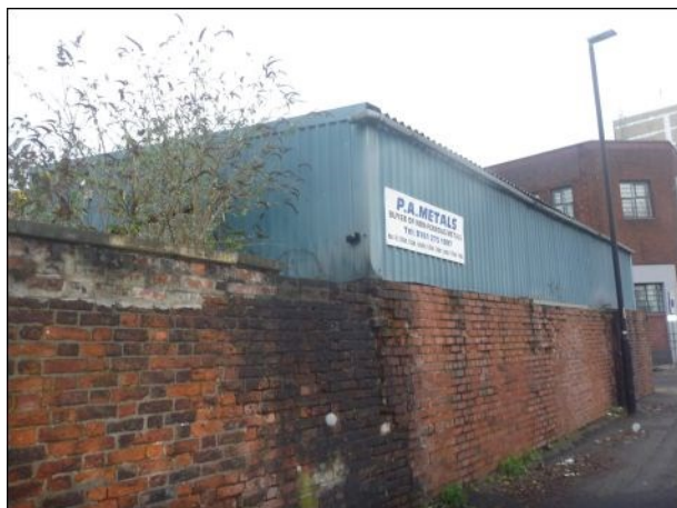
Photo 7: Building 3, south-eastern elevation
