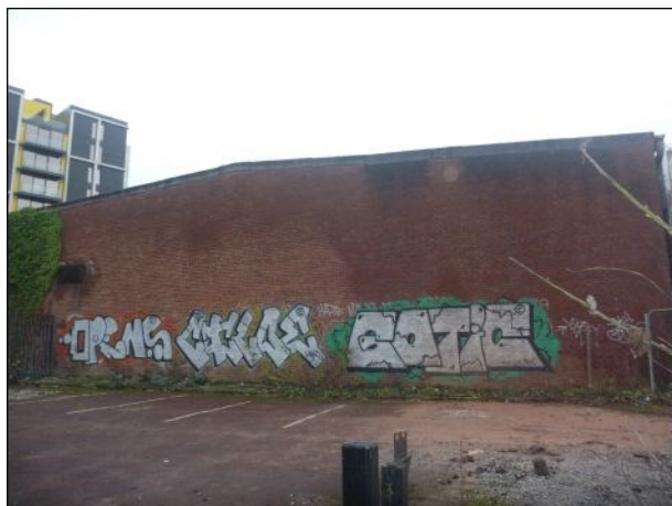
Photo 13: Building 10, south-western elevation
