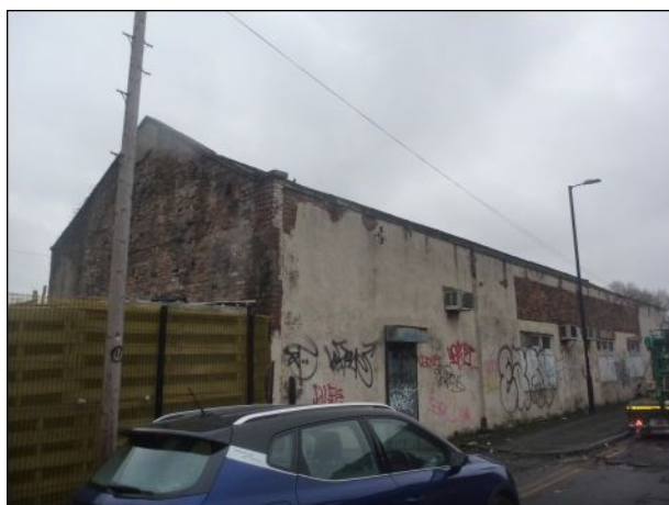
Photo 1: Building 2, north-eastern and north-western elevations
