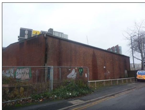
Photo 12: Building 10, south-eastern elevation
