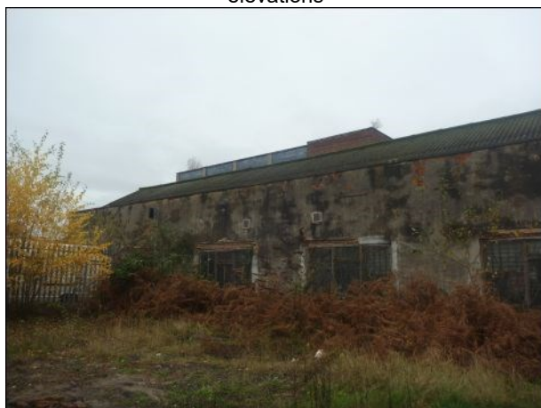
Photo 3: Building 2, south-eastern elevation
