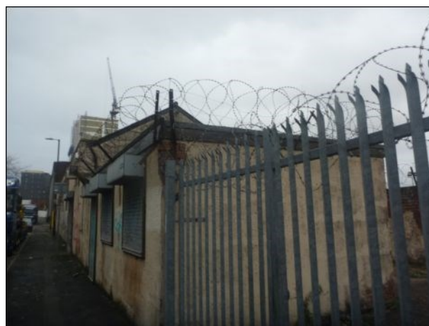
Photo 2: Building 2, south-western elevation
