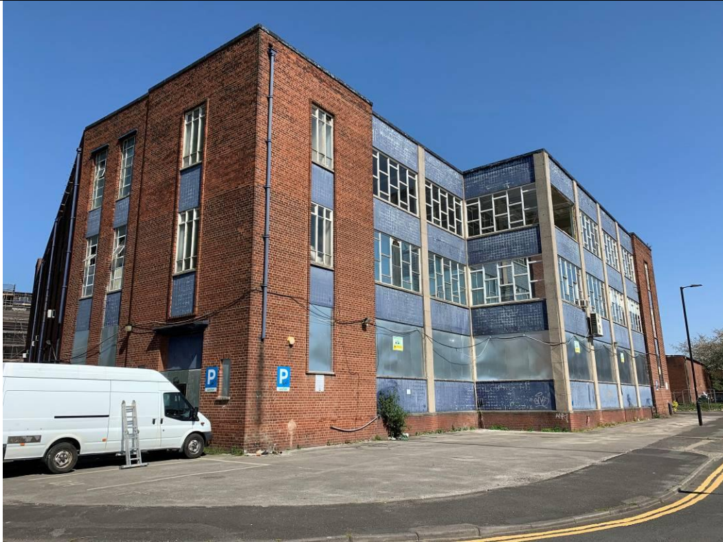
External View of the Building
