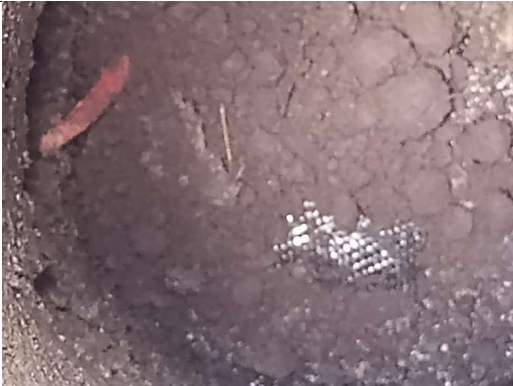
Photograph 3: Validation of Geotextile Membrane
