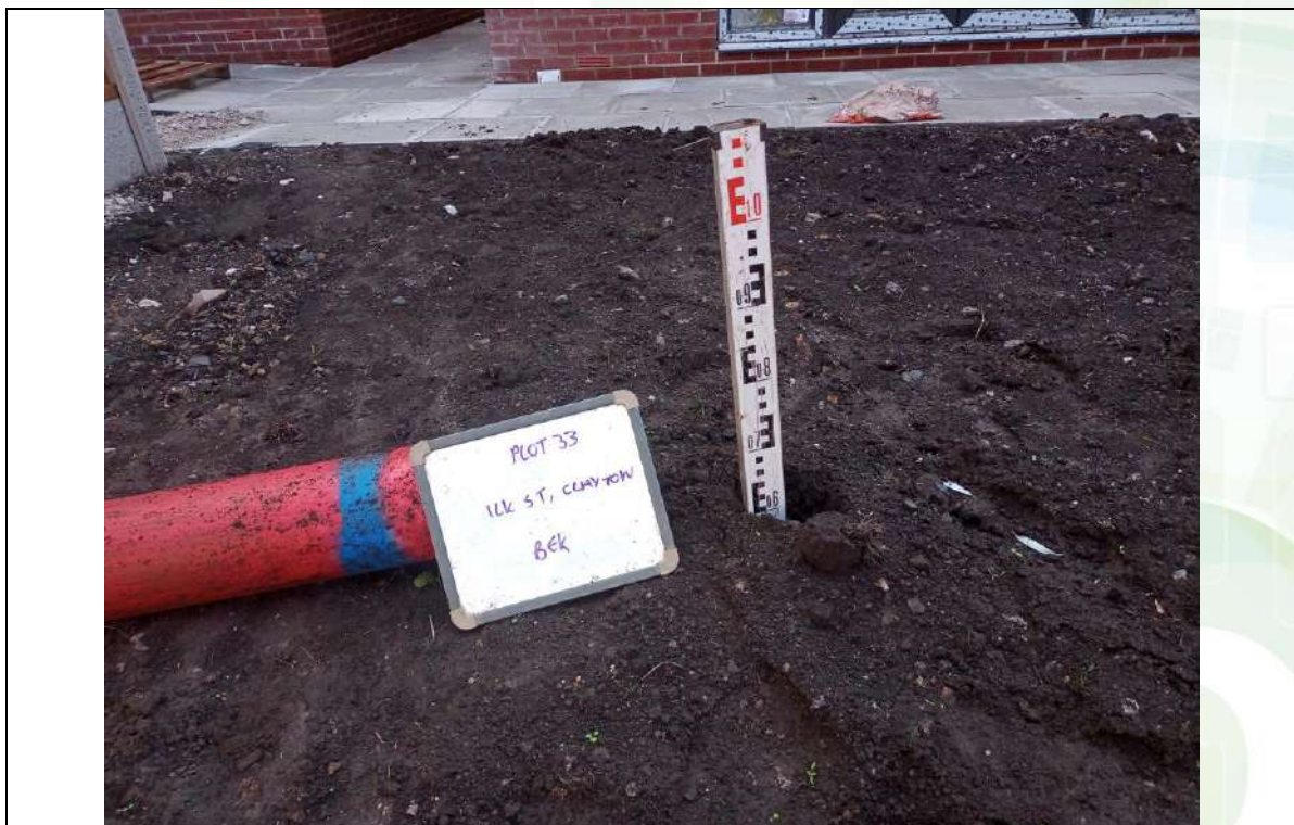
Photograph 2: Validation of Garden Capping Thickness
