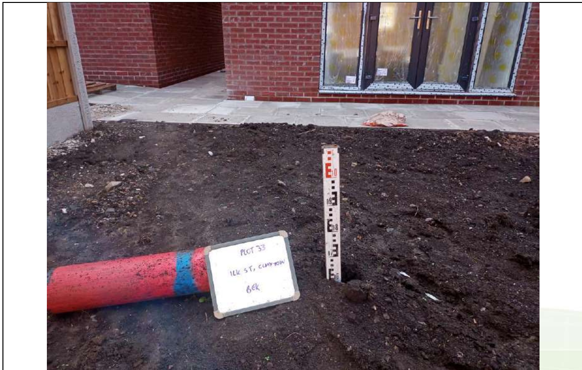
Photograph 1: Validation of Garden Capping Thickness
