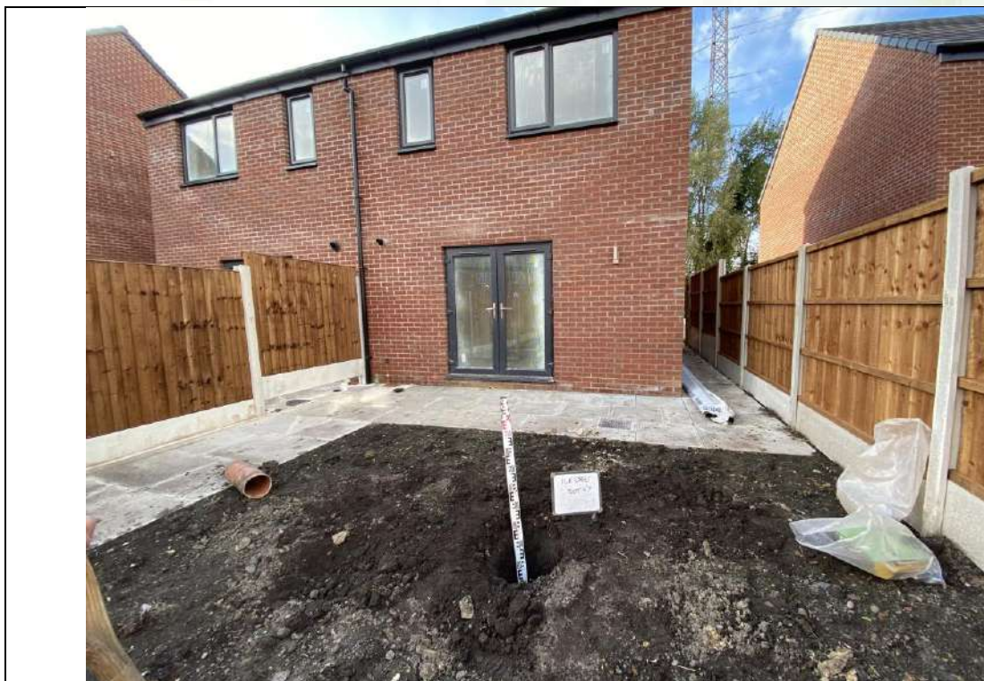
Photograph 2: Validation of Garden Capping Thickness
