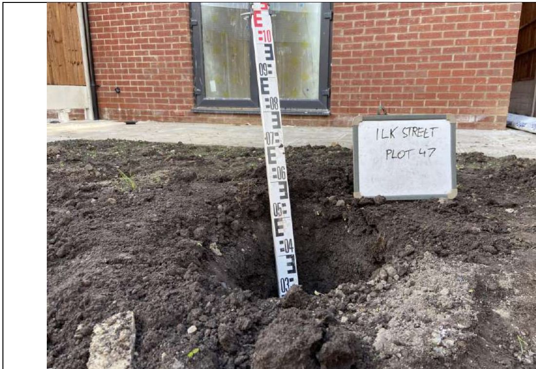
Photograph 1: Validation of Garden Capping Thickness
