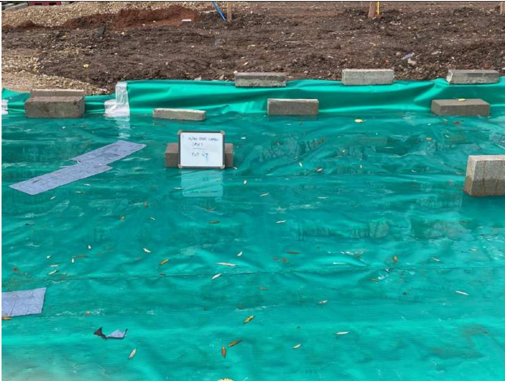
Photograph 7: Validation of Gas Membrane Installation
