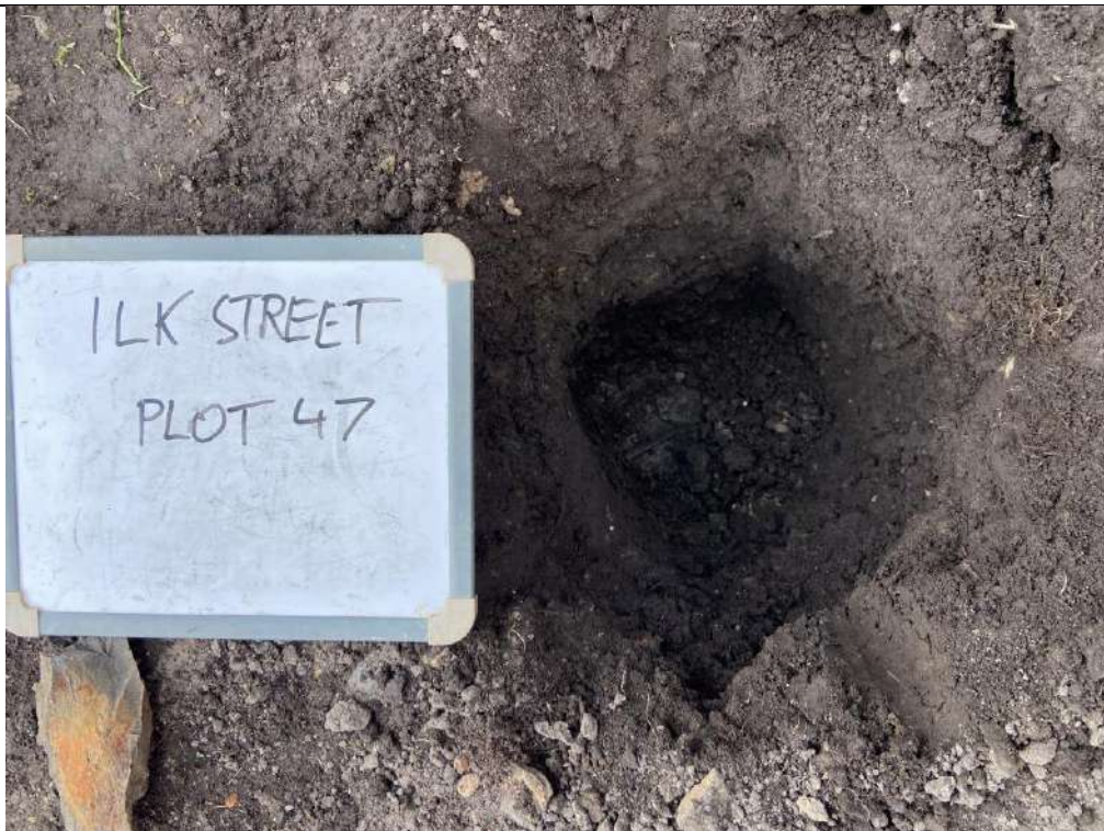
Photograph 3: Validation of Geotextile Membrane
