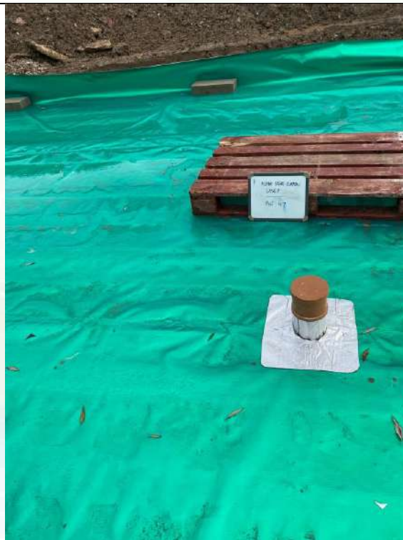
Photograph 8: Validation of Gas Membrane Installation
