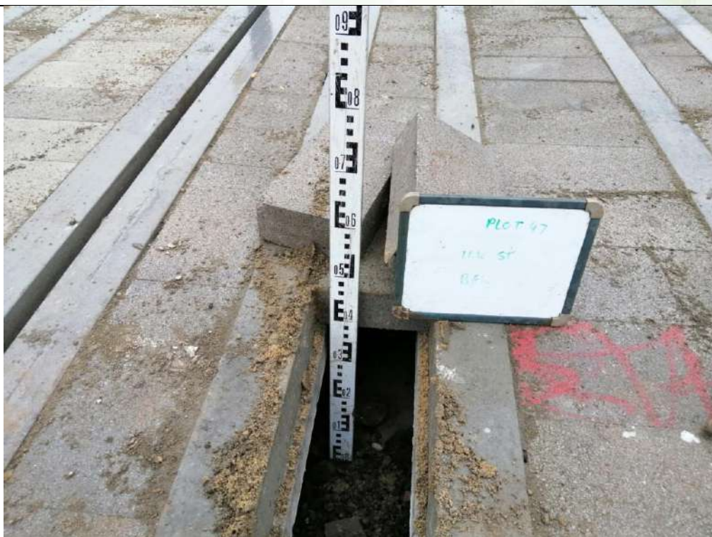
Photograph 4: Validation of Sub-Floor Void Space (min 150 mm)
