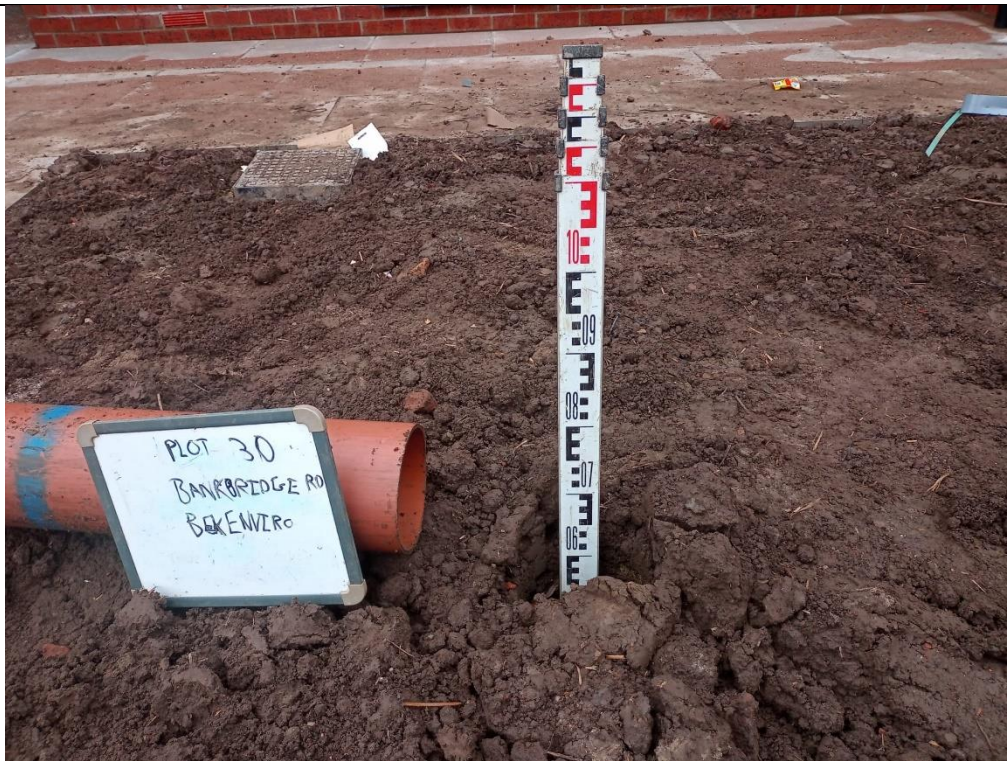
Photograph 1: Validation of Garden Capping Thickness
