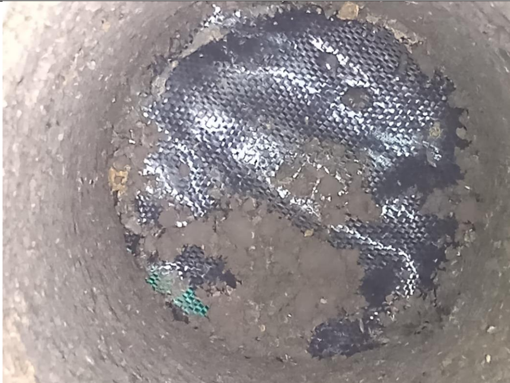
Photograph 3: Validation of Geotextile Membrane
