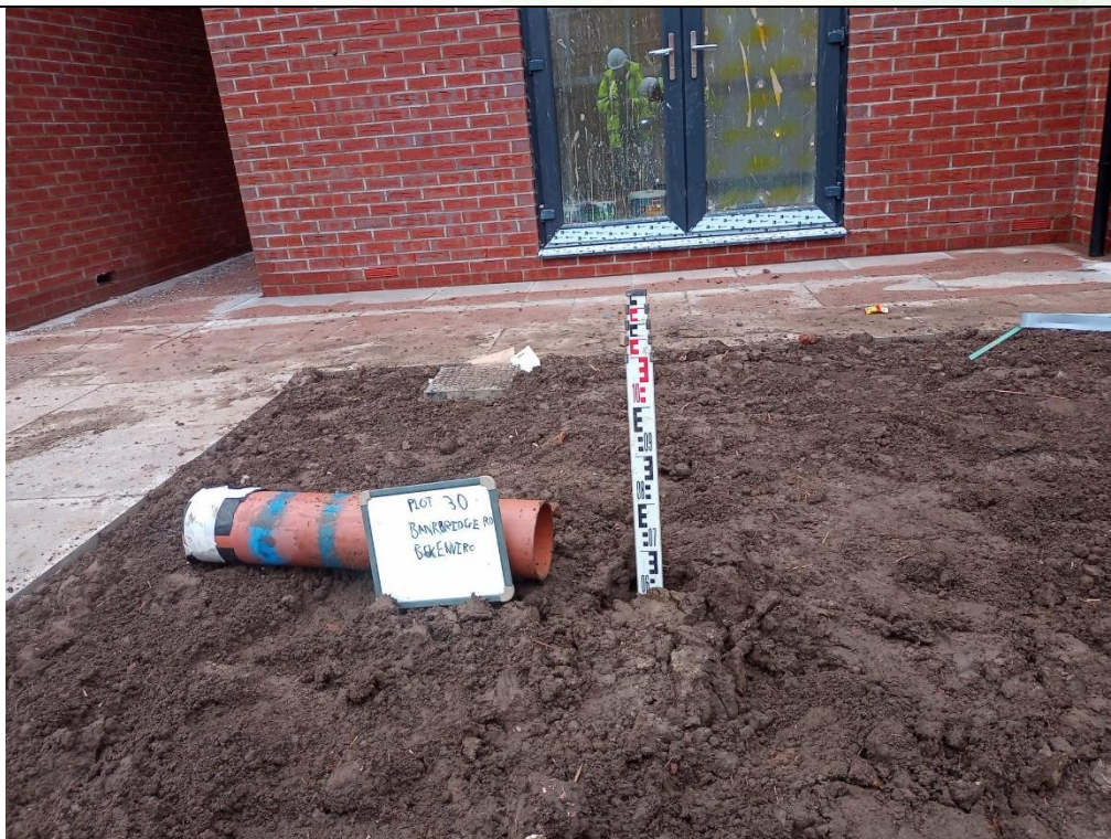
Photograph 2: Validation of Garden Capping Thickness
