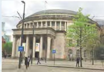
Existing - View from St Peter's Square
