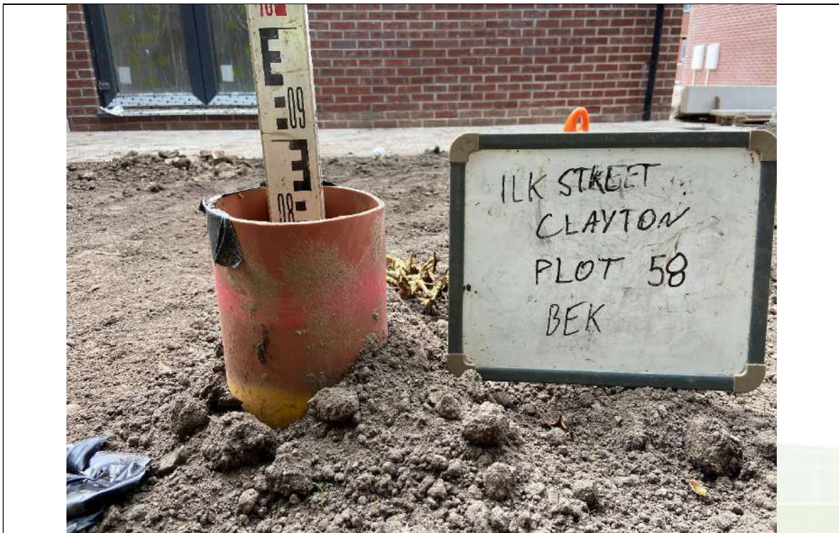
Photograph 1: Validation of Garden Capping Thickness (Plot 59, not 58)
