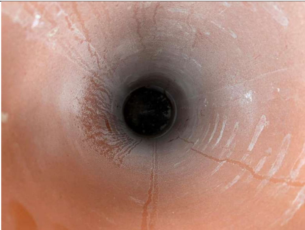
Photograph 3: Validation of Geotextile Membrane
