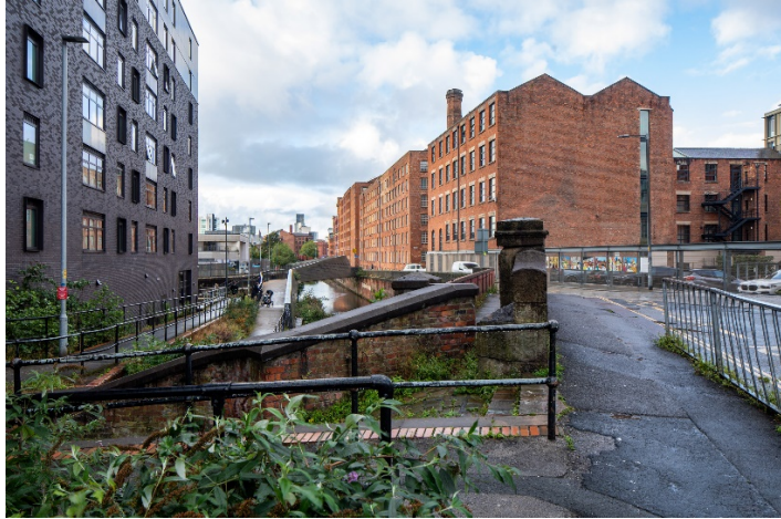
View C: Existing View
