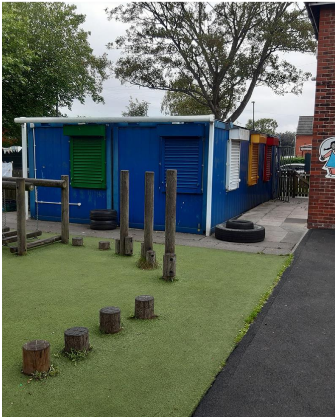
Photograph 1&2- Part South/East elevation.
