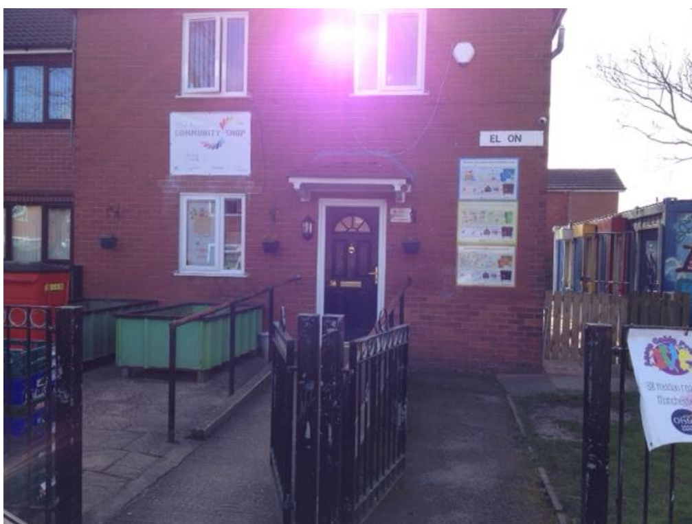
Photograph 5 -38 Meldon Road front elevation
