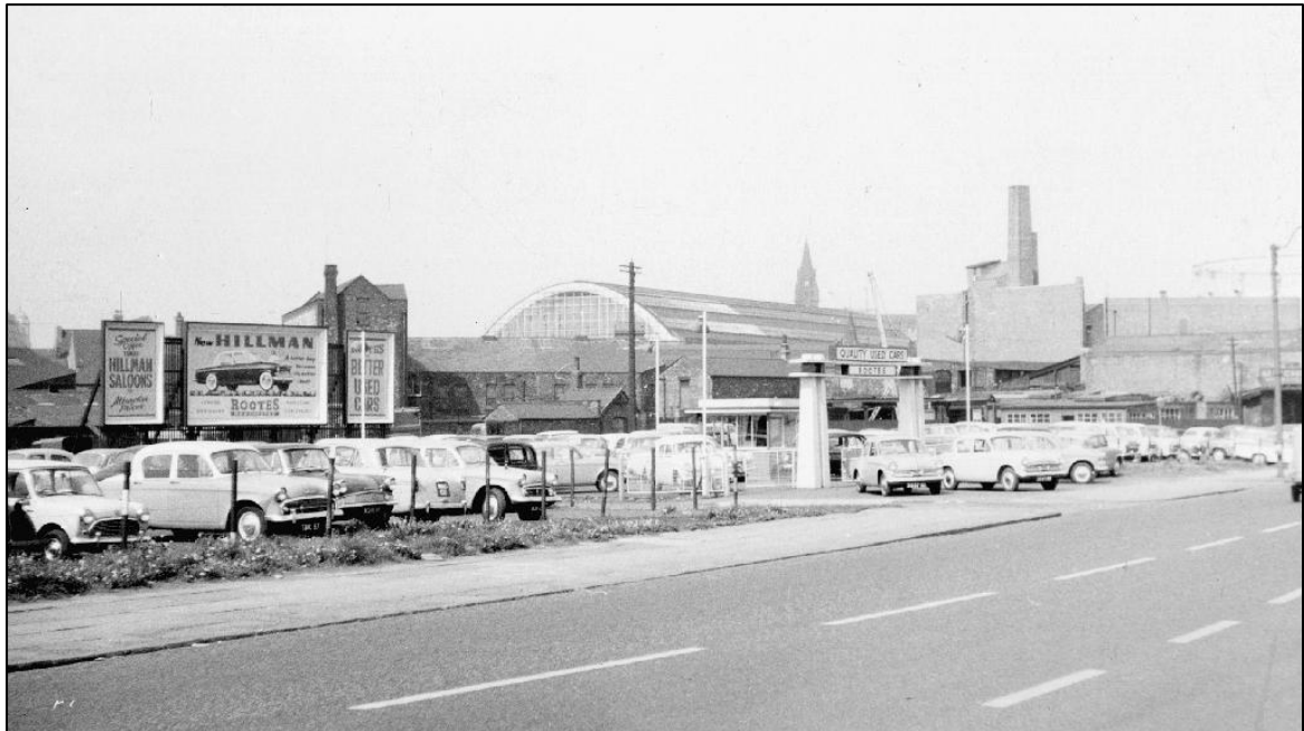
Plate 12: Site of Alpha Street and Beta Street after demolition. Hulme, 1961, looking north from City Road (now Great Jackson Street)
