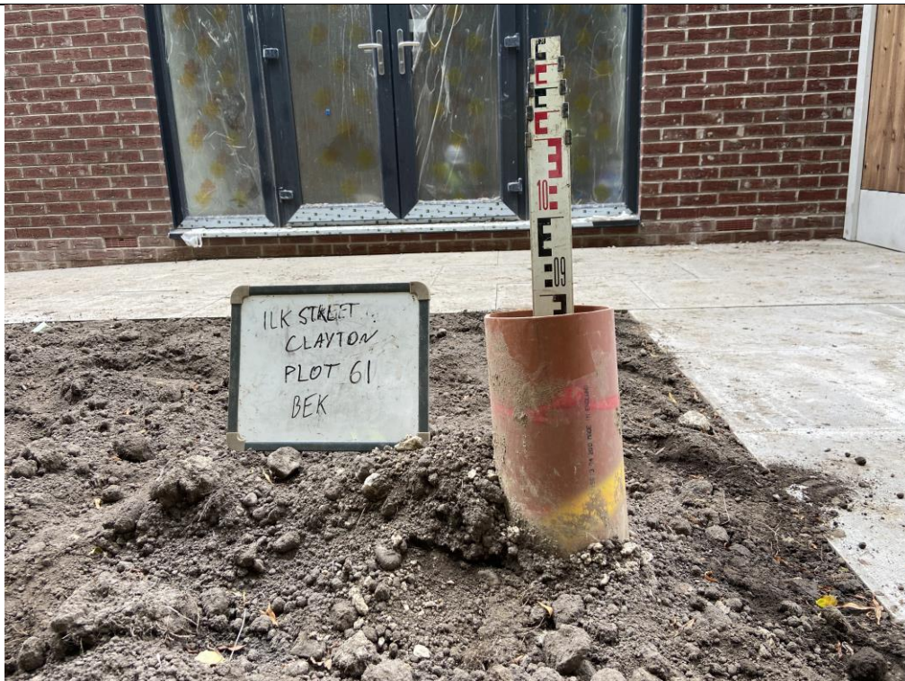
Photograph 1: Validation of Garden Capping Thickness (Plot 62, not 61)
