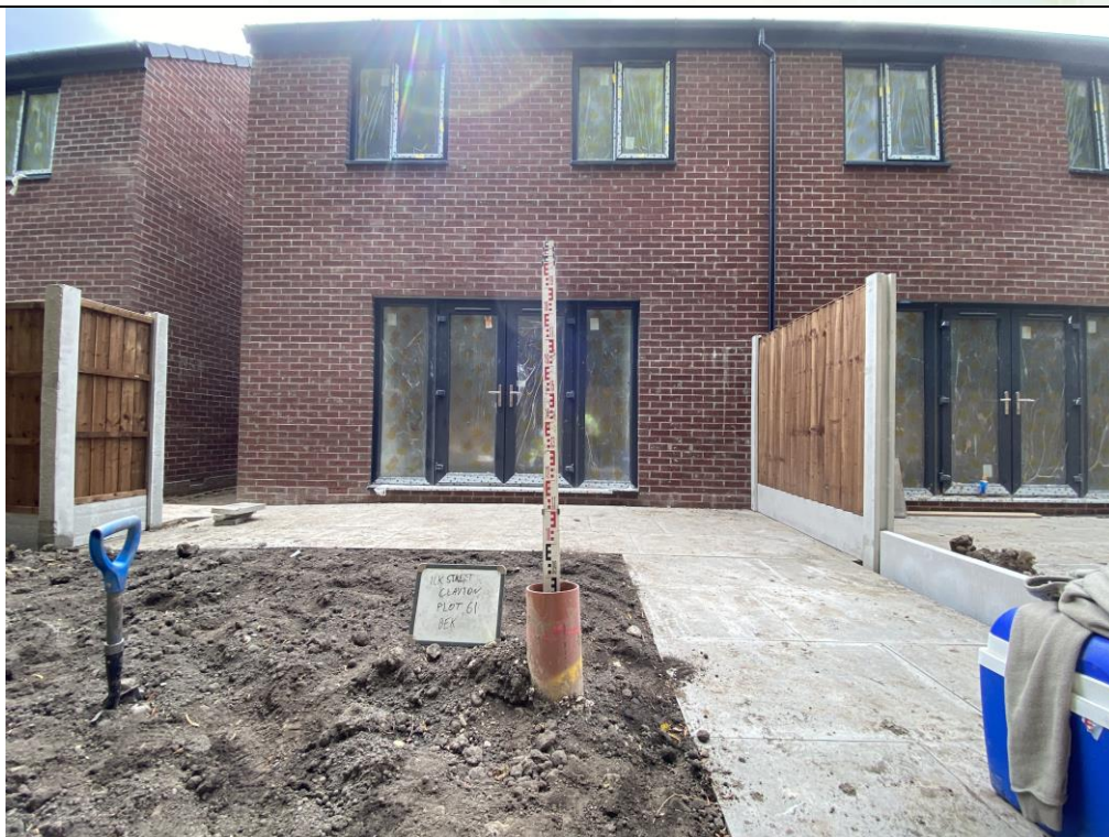
Photograph 2: Validation of Garden Capping Thickness (Plot 62, not 61)
